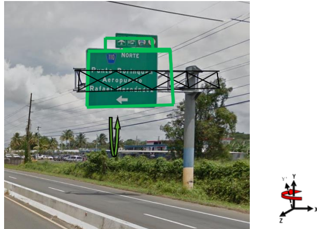
Figure 6-19: Photo of the initial CS structure position and graphical representation of rotate CS structure at Site-2. (Adapted from Google earth)
