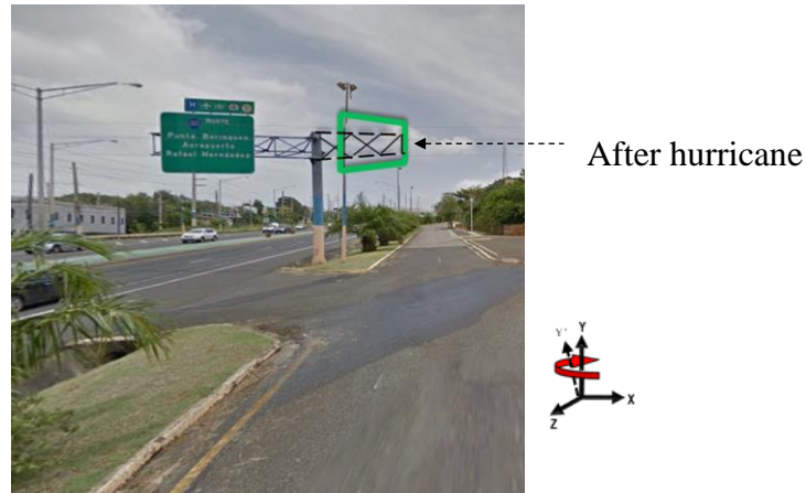
Figure 6-31: Photo of the initial CS structure position and graphical representation of rotate CS structure Site-3. (Adapted from Google Earth)
