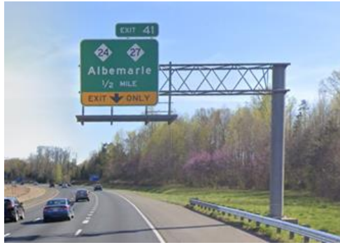
a. Photo of a cantilever sign (CS) structure and its schematic representation
