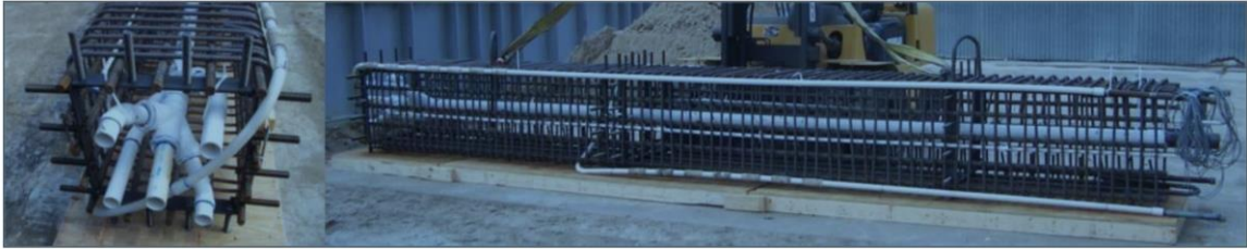
Figure 4-15: Photos of grouted precast pile reported by Herrera et al. (2017).
