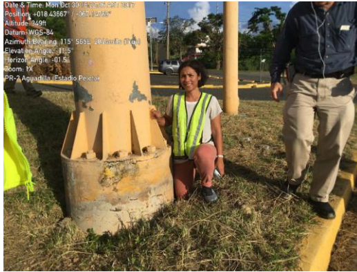
Figure 6-35: Photos of the gap between soil and DS at Site-3. FIGURE28 left (Silva-Tulla et al. 2018)
