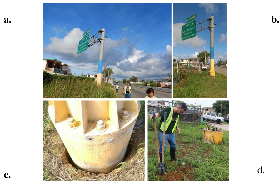
Figure 6-4: Photos of CS structure rotated after hurricane Maria at Site-1. Figure 6-4(a) (Silva-Tulla et al. 2018)
