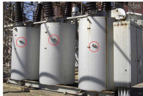
Figure 6.2.b: Oil-filled circuit breakers in TVA's Paradise substation. The wireless sensor nodes that sense the surface temperatures are marked by red circles
