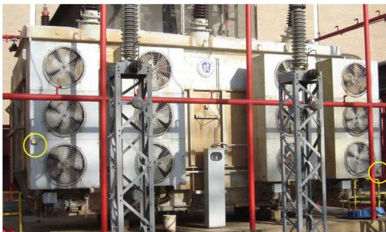
Figure 6.2.a: An oil-cooled transformer in TVA's Paradise substation, showing two wireless sensors marked by yellow circles
