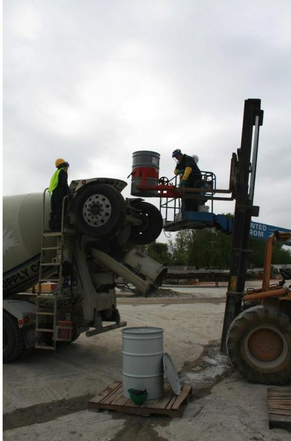
Figure: 2.6 Activating solution pouring into concrete mixing truck.
