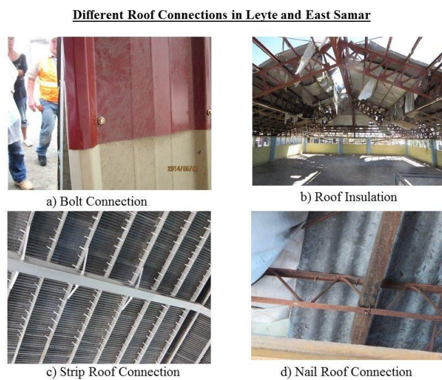
Figure 34: Different Roof Cover Connections in Leyte and East Samar Islands
