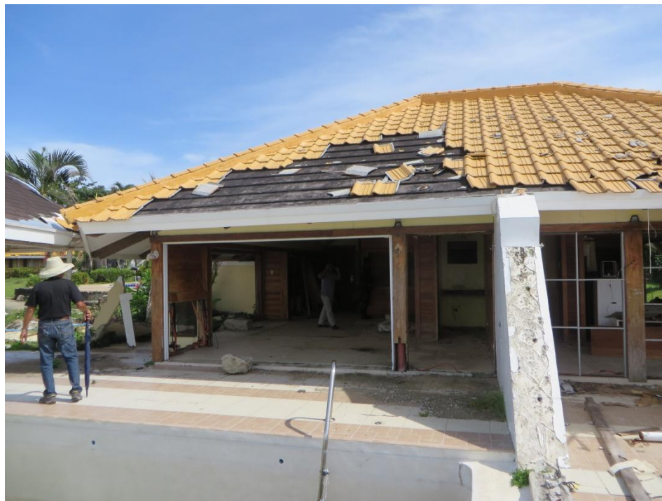
Figure 32: Storm Damaged Metal Roof (B01-003-013)
