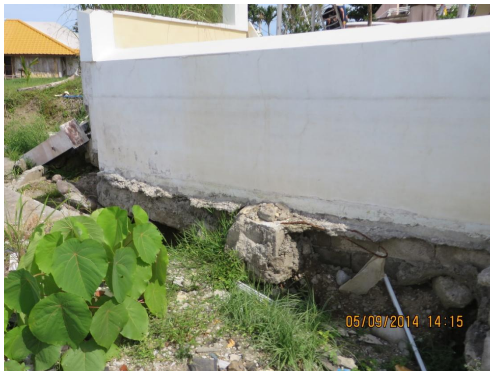
Figure 28: Severely Scoured Foundation (B01-003-013)
