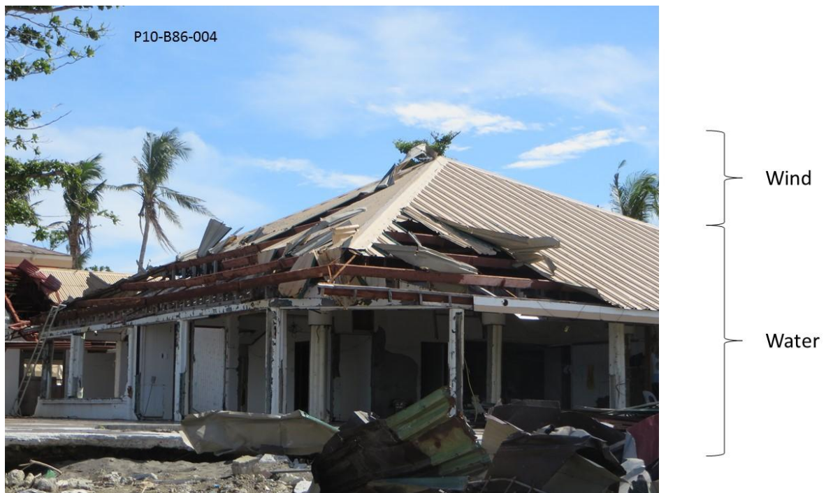
Figure 26: One-Story Residential Structure (P10-B86-004) with Wind and Water Damages
