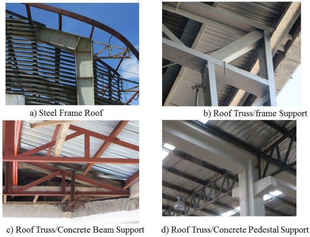
Different Roof Support Systems in Leyte and East Samar
