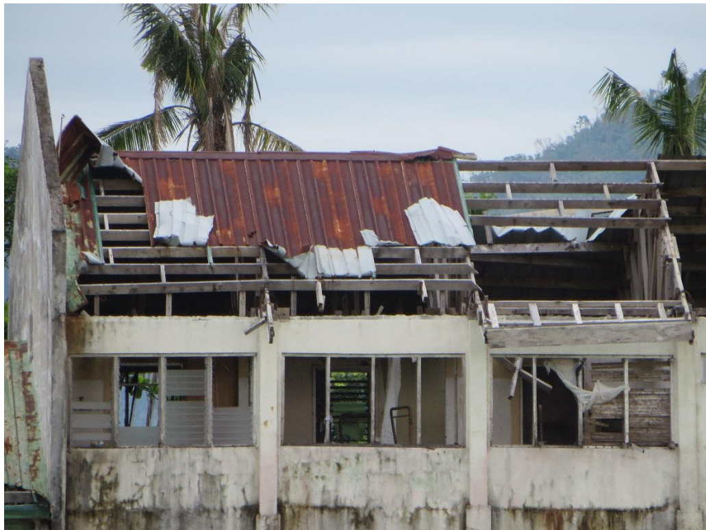
Figure 24: Damaged Two-story Structure (B88-030) near Tacloban Domestic Airport Depicting Metal Roof Panels, Wood Truss and Reinforced Concrete Walls
