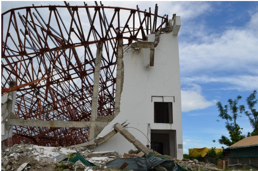
Figure 30: Roof Truss Connection for the Commercial Structure (Palo-008-D2)
