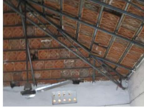
b) Truss and Frame Support for Tile and Shingle Roofing
