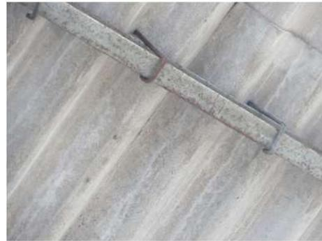
d) Hook Connection of Sheet Metal Roofing
