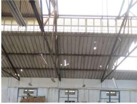
a) Tubular Truss Roofing System for Metal Sheet Roofing
