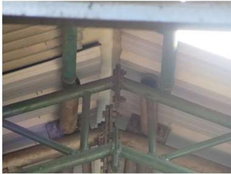
c) Bolt Connection for Roof Truss Support
