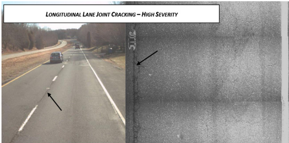
FIGURE 5: Longitudinal lane joint cracking (NCDOT, 2011)
