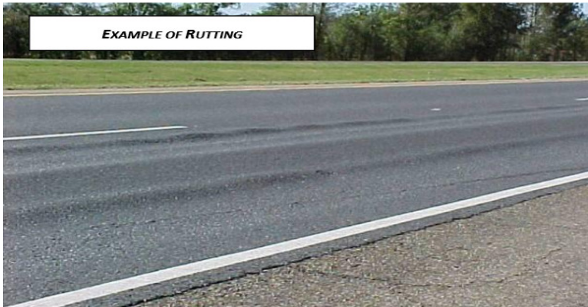
FIGURE 7: Rutting (NCDOT, 2011)
