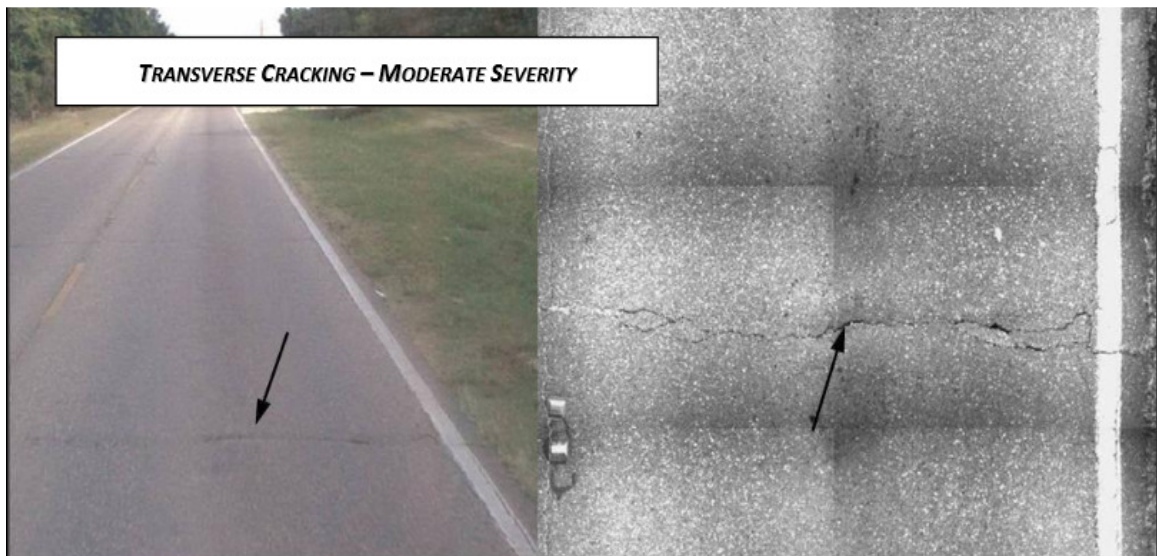
FIGURE 3: Transverse cracking (NCDOT, 2011)
