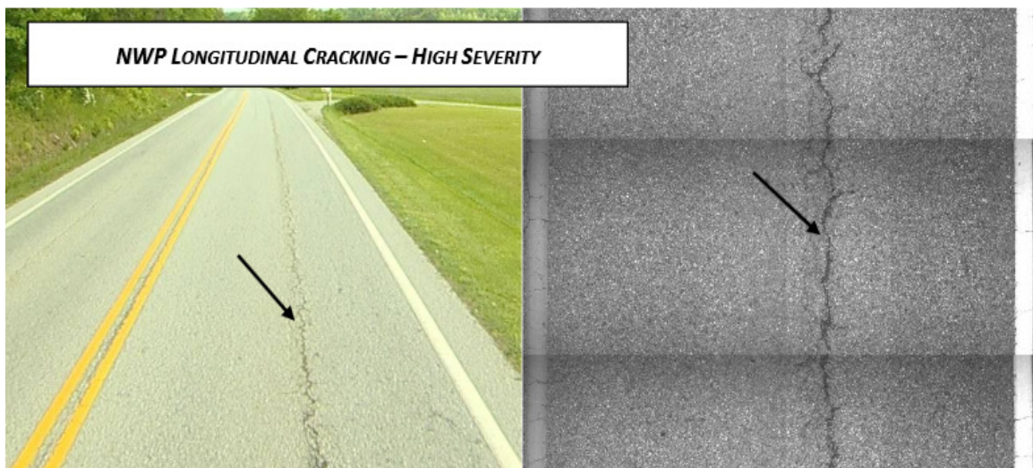
FIGURE 4: Longitudinal cracking (NCDOT, 2011)
