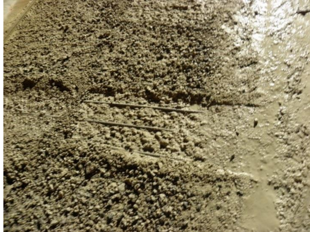
FIGURE 2: Post-hydrodemolition surface
