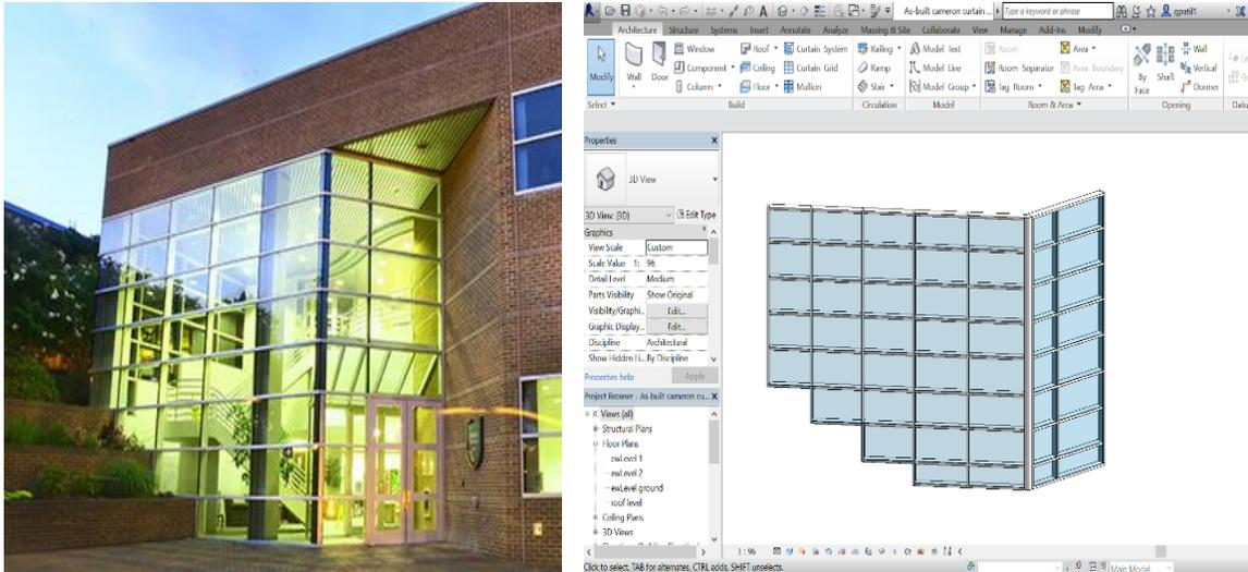
FIGURE 8: Cameron Curtain wall: Actual wall vs as-built model
