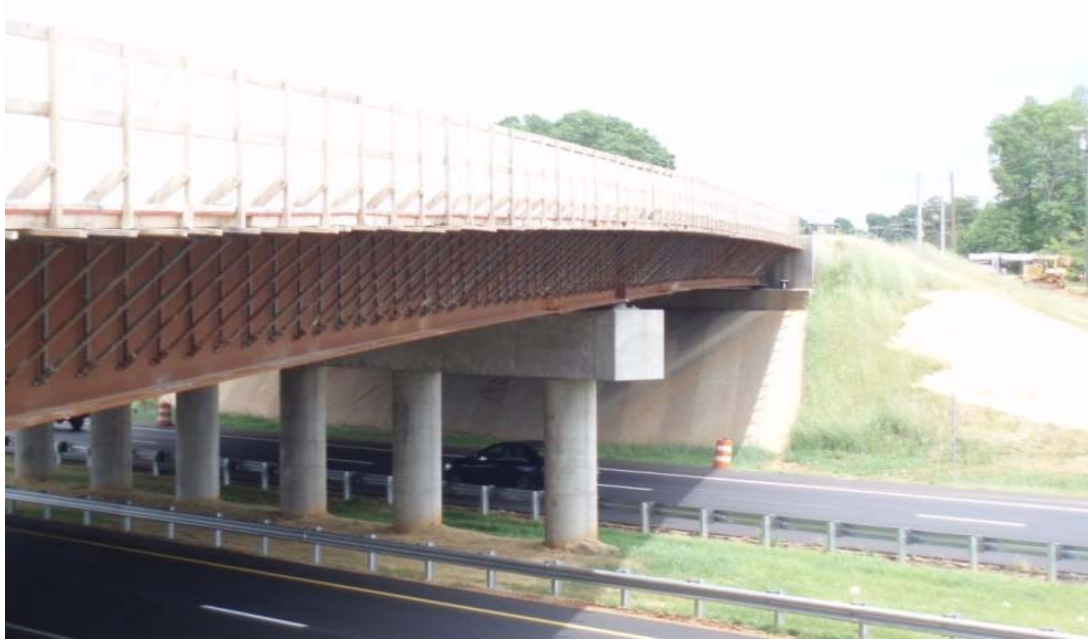
Figure 5-2 Digital photo of the Hybride HPS Bridge on Langtree Rd (SR1102) over I-77
