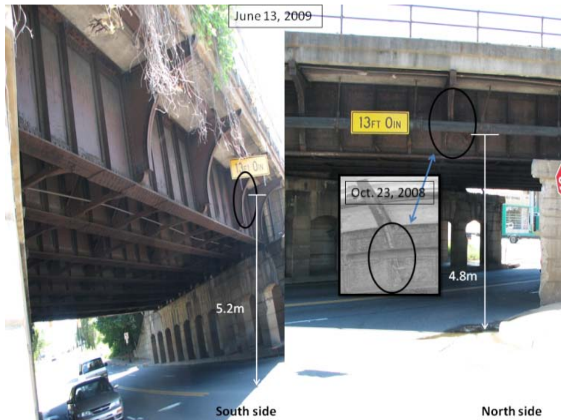
Figure 4-31 Height of collision damage location for Bridge # 590700
