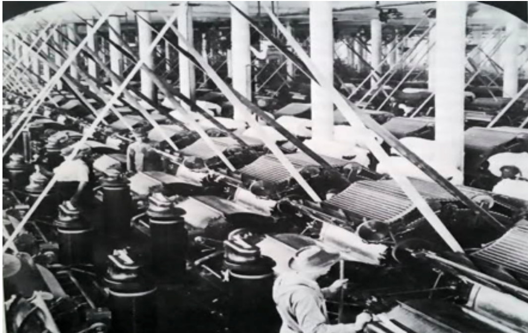
Figure 4: The Carding Machines. Noticed the pulley belts extending to the ceiling, this was the most dangerous part of working cards.
