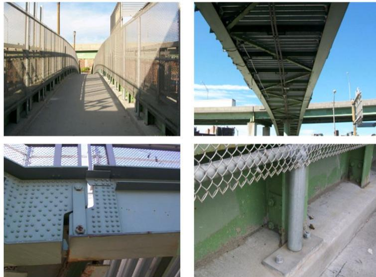
FIGURE 3.5: Bridge deck (top left). Bridge framing (top right). Pin and hanger assembly (bottom left). Girder stiffener (bottom right).
