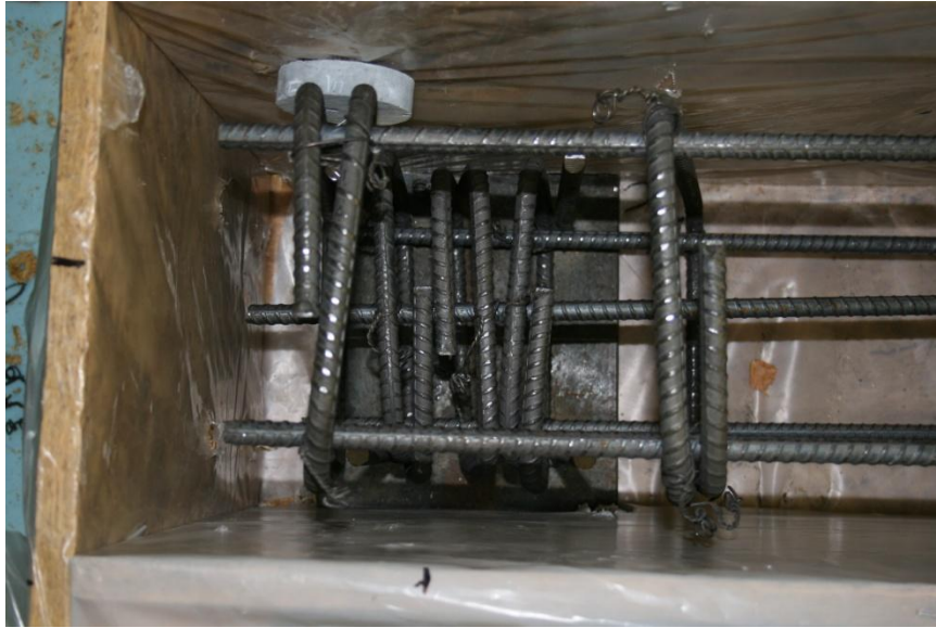
FIGURE 4-20: Extra reinforcing near the end of the prestressed beams.
