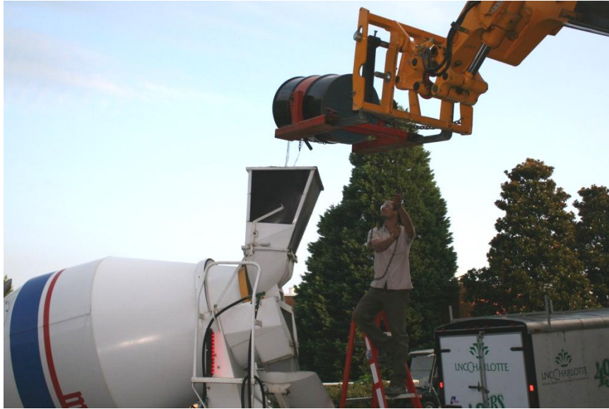
FIGURE 4-1: Adding materials to mixing truck.
