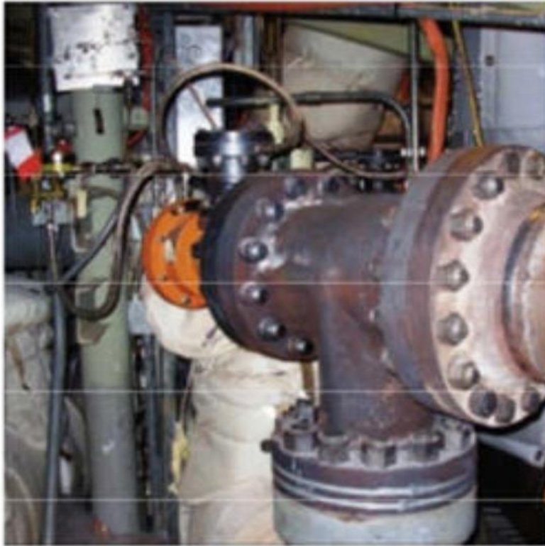
Figure 40. A safety relief valve Reactor core isolation cooling system
