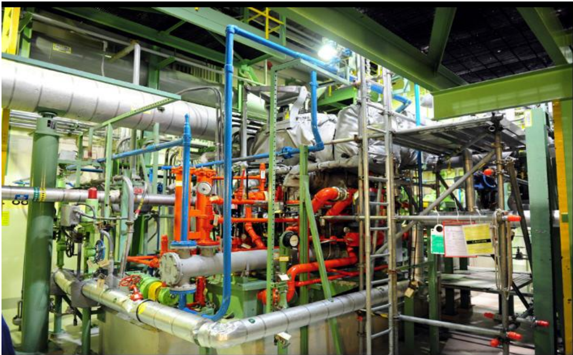
Figure 31. An image of a high-pressure coolant injection turbine [76]
