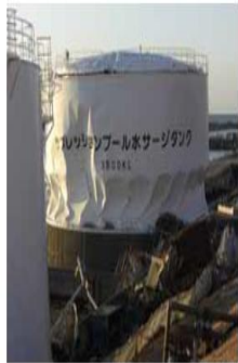
Tank deformed by the tsunami (Same tank shown in picture above)
