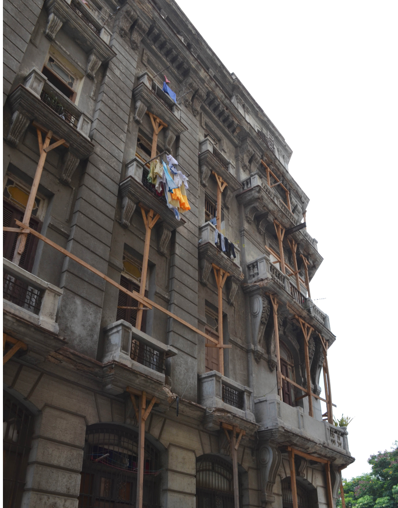
FIGURE 1: Wooden scaffolding frequently supports structurally failing balconies. The laundry hanging outside indicates that these homes are still occupied and the balconies are in use. Photograph by author.
