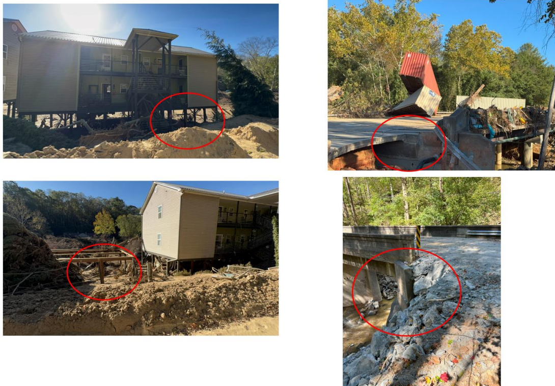
Figure 4-6 Scour (red circle) of building and bridge foundations in Asheville region. (Photo Credits: Shen Chen and Sophia Lin)
