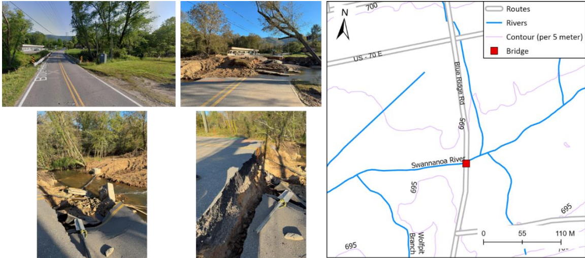
Figure 4-21 Collapsed bridge (ID: 100041) washed out by Hurricane Helene flooding. (Photo Credits: Sophia Lin and Shen Chen)
