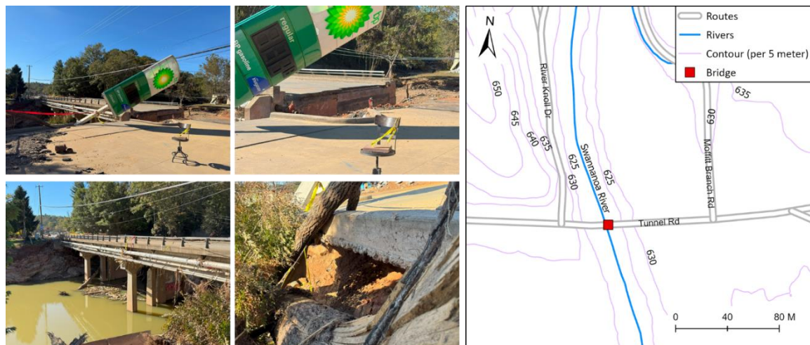
Figure 4-16 The Tunnel Road Bridge (ID:100239) over Swannanoa River in Asheville, NC, experienced support mass loss at the bridge approach after Hurricane Helene. (Photo Credits: Sophia Lin and Shen Chen)
