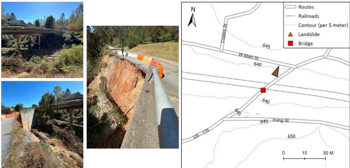
Figure 4-18 Damaged I-176 Bridge on Main Street, Saluda, North Carolina (The damage to the bridge abutment is due to a debris slide around the wing wall). (Photo Credits: Sophia Lin and Shen Chen).
