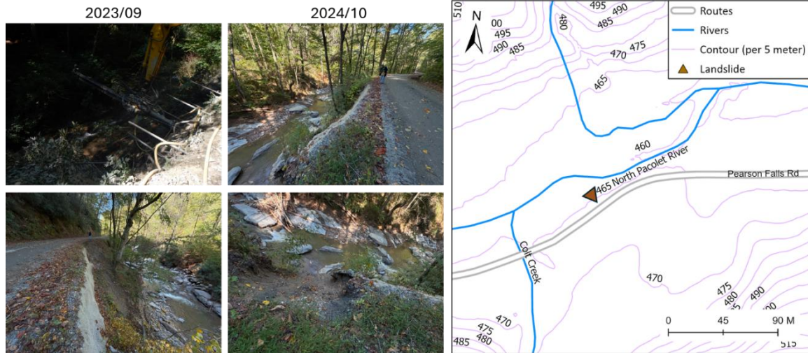
Figure 4-13 Landslide at a previously grouted and repaired slope. (Photo Credits: Sophia Lin and Shen Chen)
