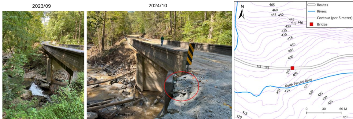
Figure 4-15 Bridge (ID:740027) on highway 176 experienced support mass loss at the bridge approach after Hurricane Helene. (Photo Credits: Sophia Lin and Shen Chen)
