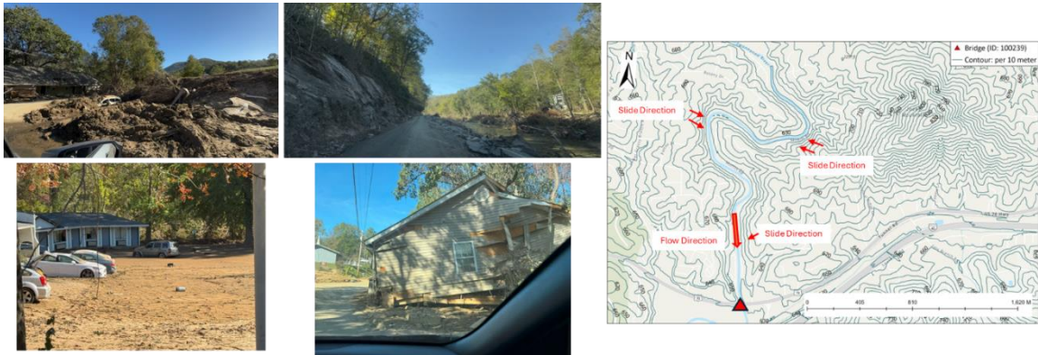
Figure 4-17 Massive debris filled floodwater resulted in mud caked cars and lots and damaged buildings and constricted the Swannanoa River, Asheville, NC. (Photo Credits: Sophia Lin and Shen Chen)
