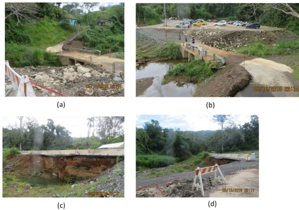
Figure 2-4. A new bridge under construction in Las Marias - Heavy flooding resulted in localized landslides and the washout of the original bridge. (Photo credit: Shen-En Chen)
