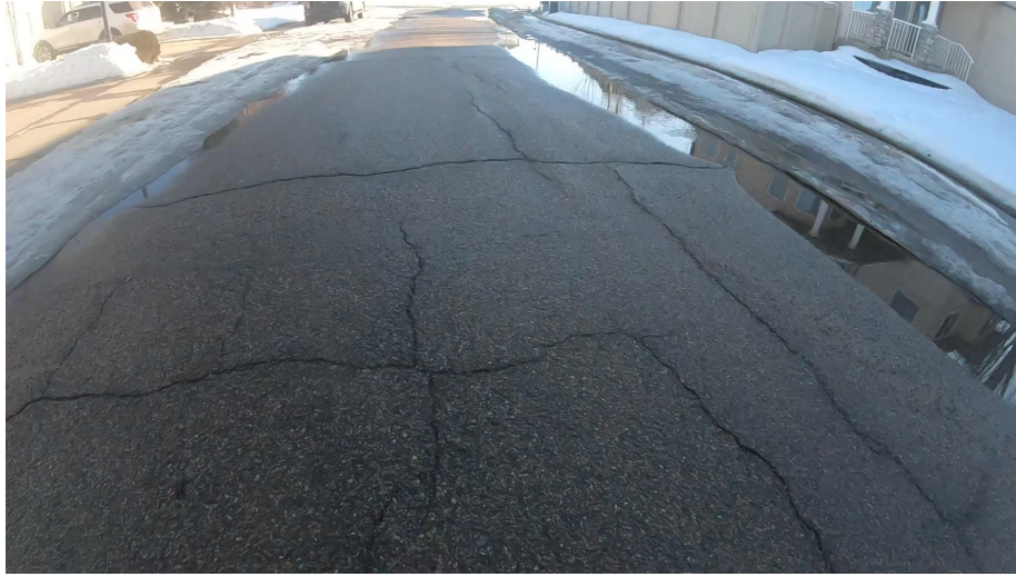
Figure 7. Alligator crack - moderate severity, source: [3]
