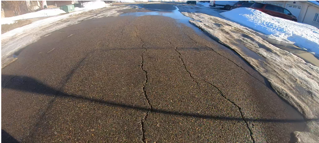
Figure 27. Exceptional alligator crack with low severity, source dataset: [3]
