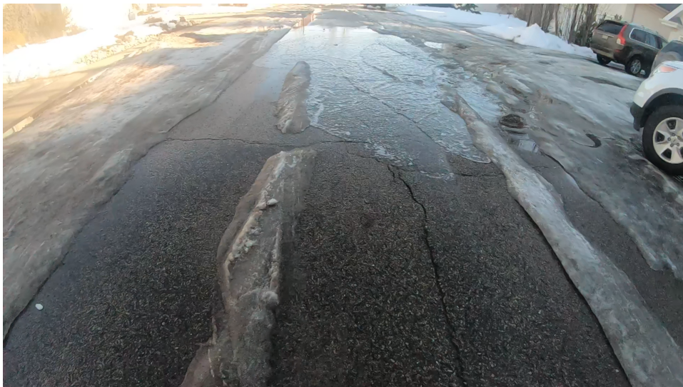
Figure 6. Alligator crack - low severity, source: [3]
