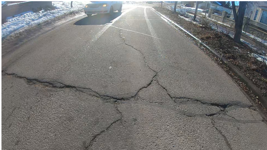
Figure 8. Alligator crack - high severity according, source: [3]
