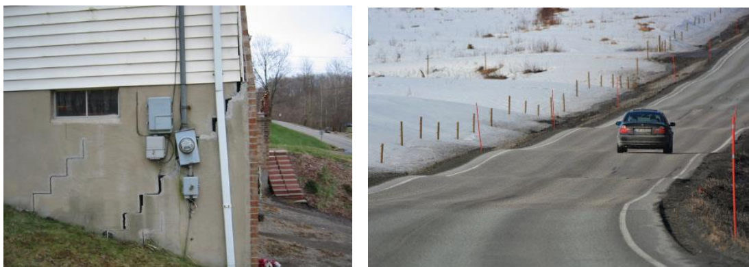
Figure 0-2 Frost heave damage to foundations (ECP, 2011) and roadways (Ystenes, 2013)
