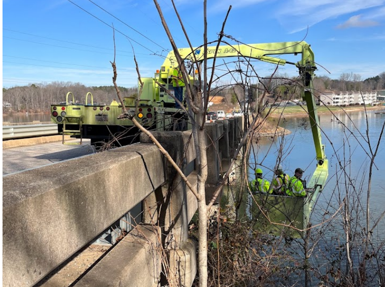
Figure 10: Inspectors Performing Bridge Inspection in a Snooper Truck
