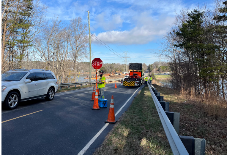
Figure 12: Traffic Control Setup During an Inspection Operation
