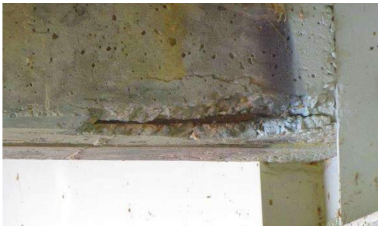
Figure 15: Typical Spall in Concrete
