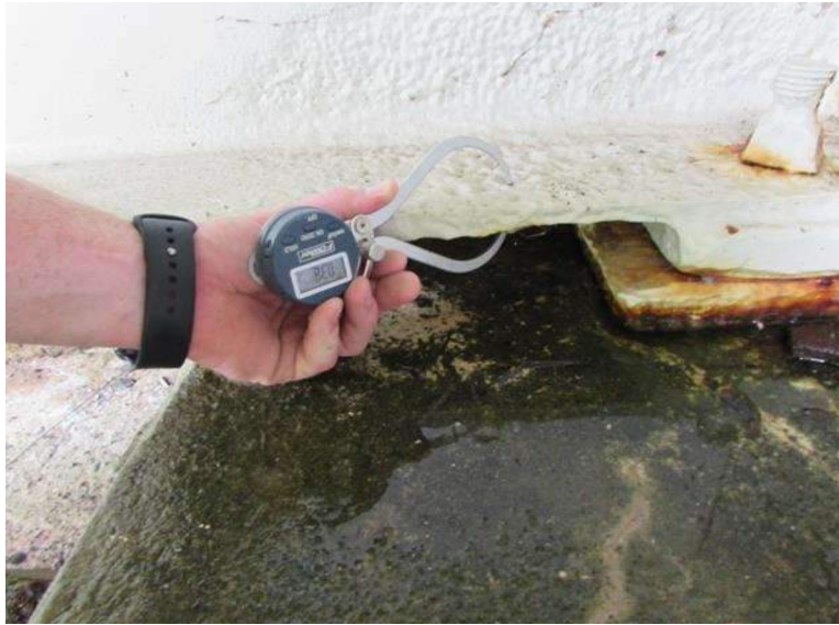
Figure 17: Typical Corrosion on a Steel Member
