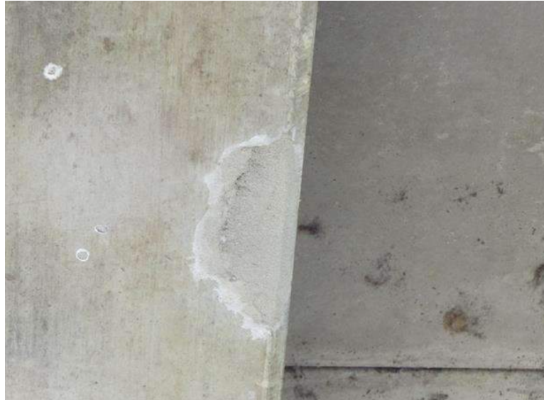
Figure 16: Typical Patch in Concrete
