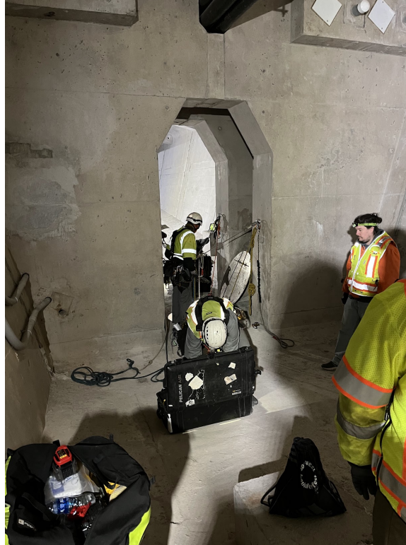
Figure 9: Regular Inspection Team and Ropes Team Performing Bridge Inspection Inside a Box Girder
