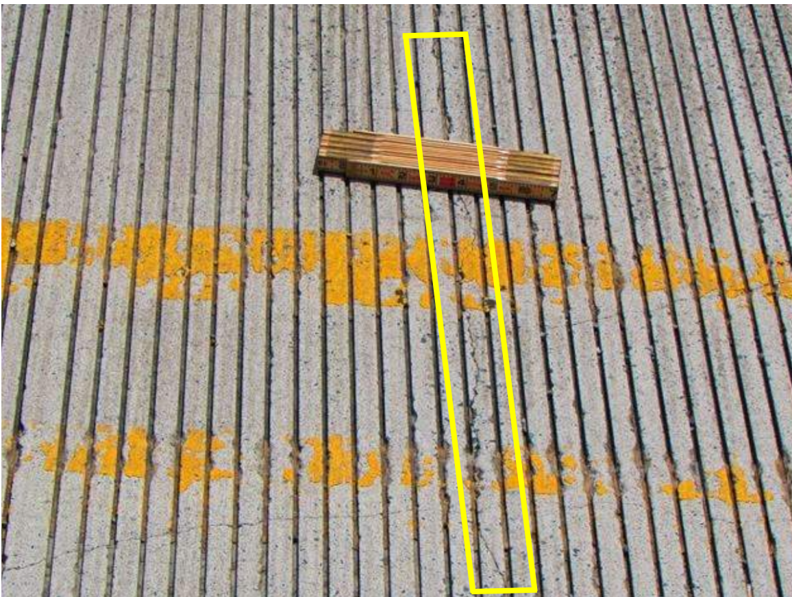
Figure 14: Concrete Hairline Crack
