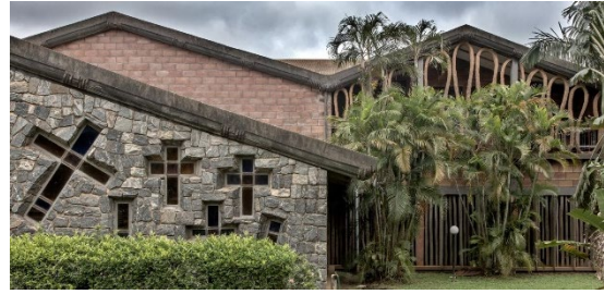
Figure 14. The Dominican Institute's lounge and refectory feature stone, bamboo screens, brick and sand-casted screen walls. The latter provide both natural ventilation and large-scale decoration [94].
