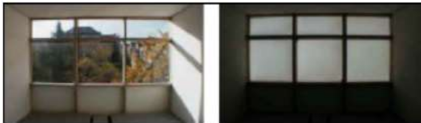
Figure 9: Effect of temperature and light diffusion through thermotropic glass[23]
