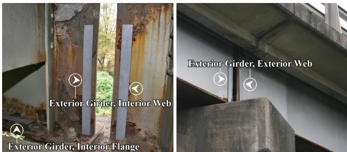
FIGURE 4.3: Coupons placement and location for atmospheric exposure
