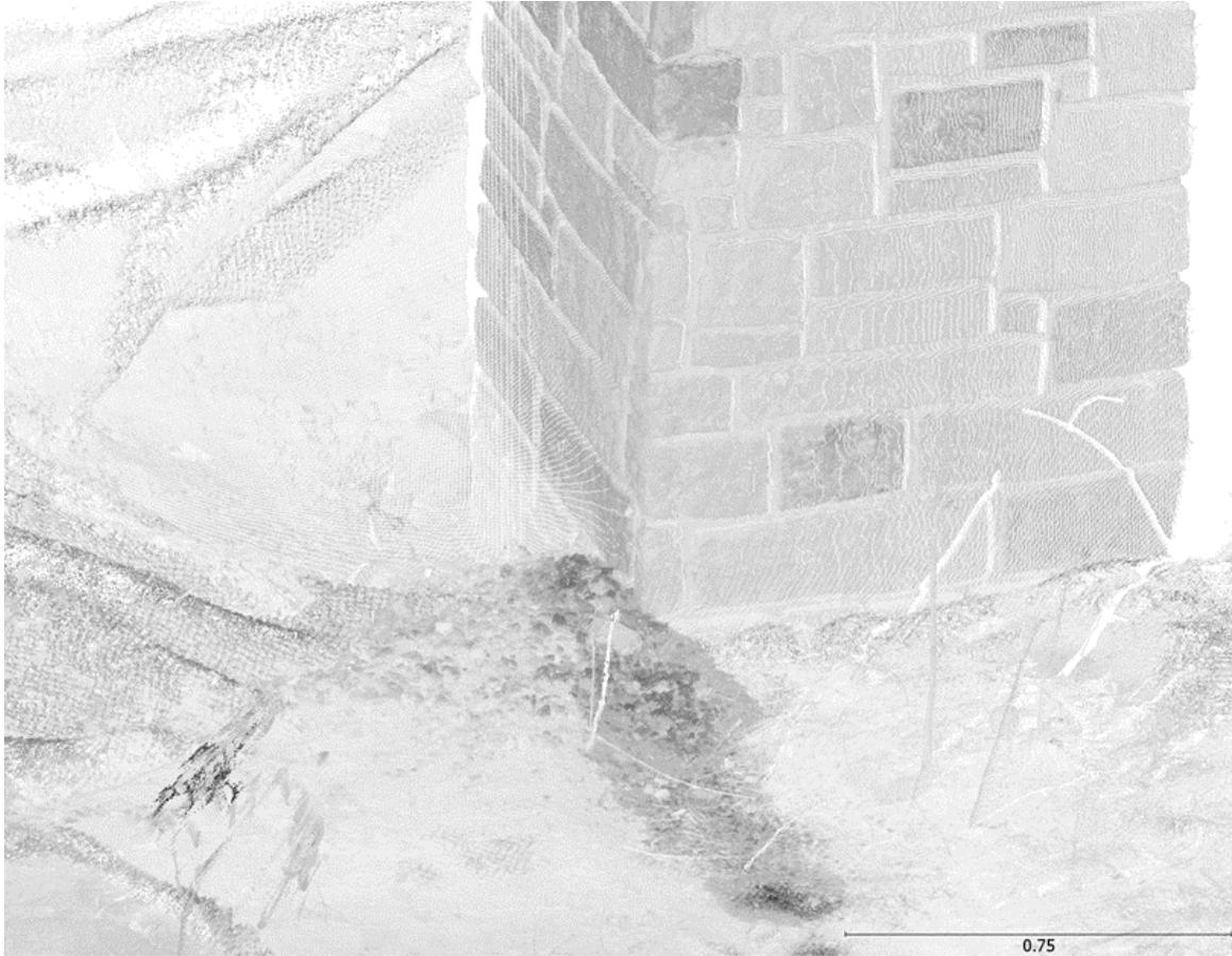
Figure B-1 Point cloud of Phillips Road Bridge North Bank Pier No. 2 and scour as on Feb 11, 2019
