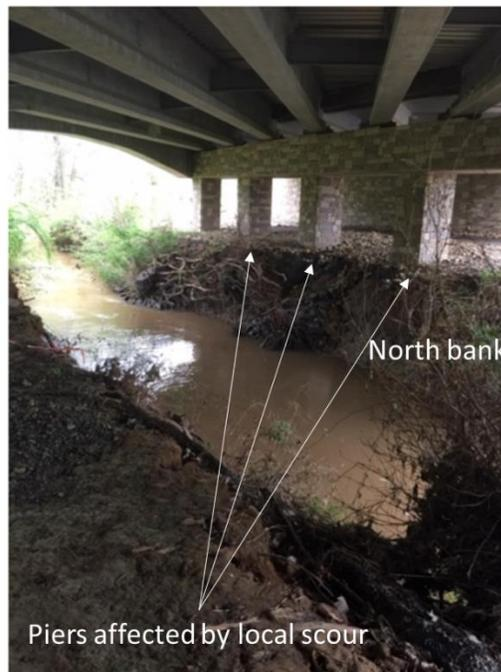
Figure 3-3 Snapshots of Phillips Road Bridge (on 03/30/2019)
