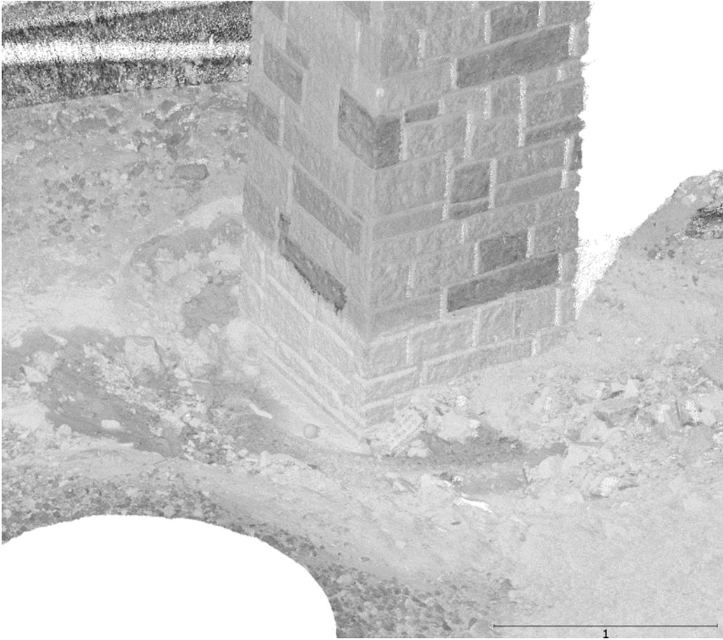
Figure C-1 Point cloud of Phillips Road Bridge North Bank Pier No. 3 and scour as on Aug 17, 2019
