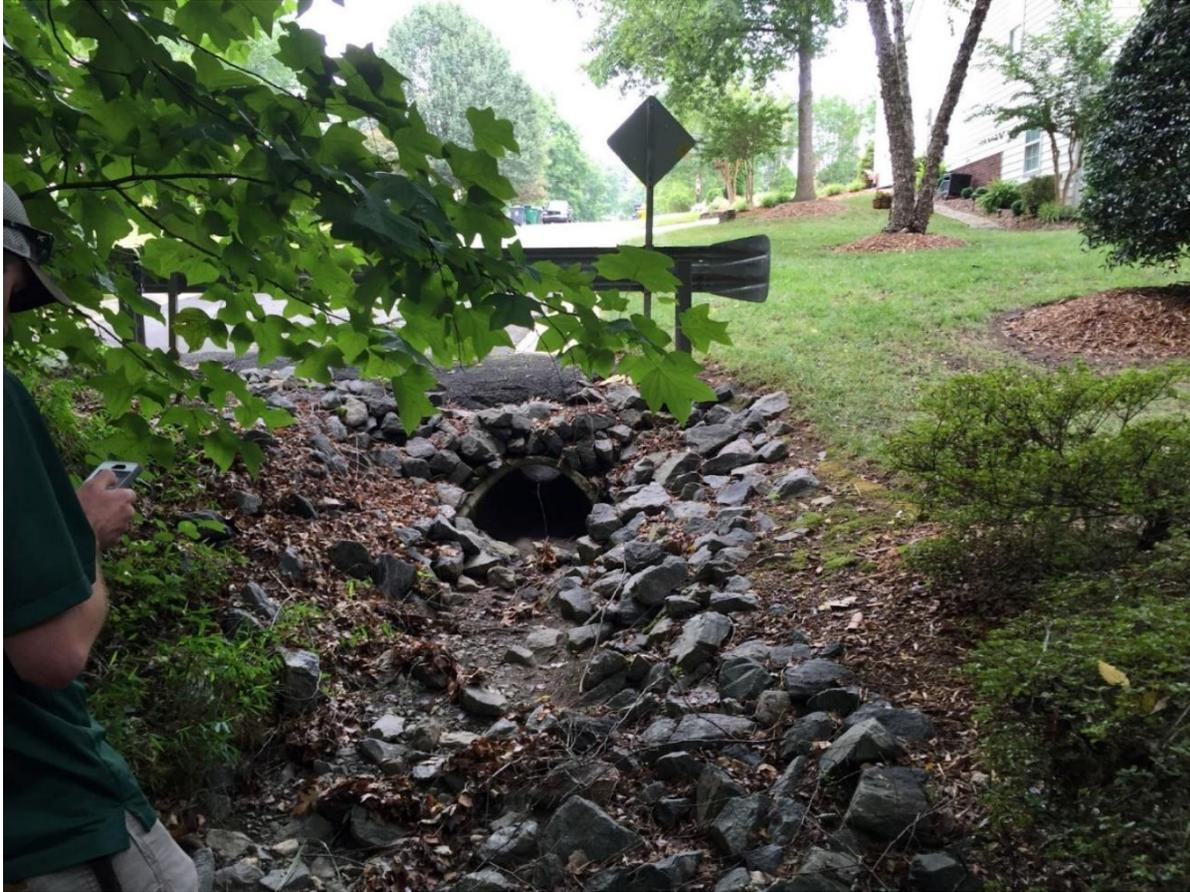
**Figure 4.4.** Storm drain located at the upper end of site I1 on the stormwater impacted tributary (TI).
