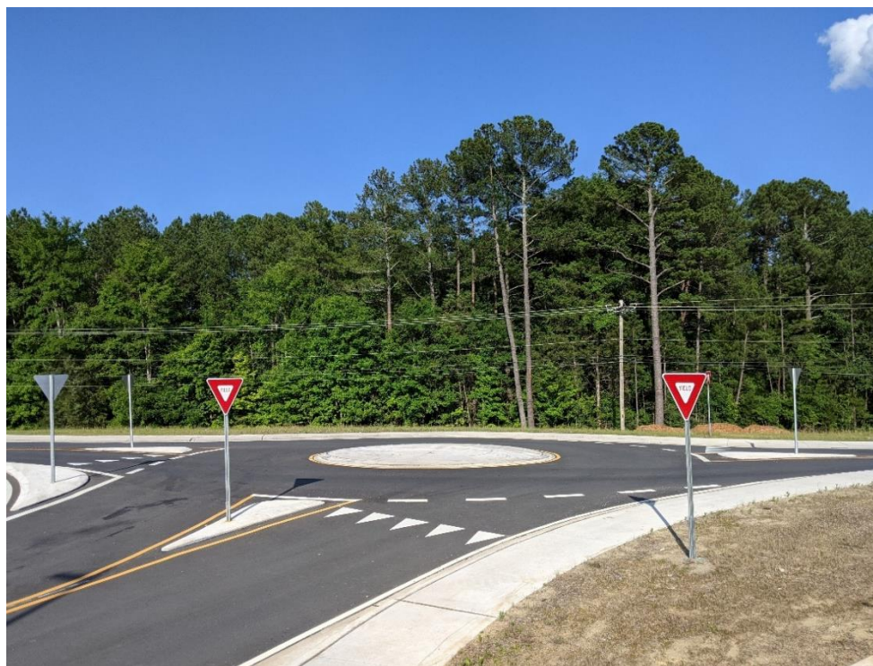
Figure 3-4. Mini-roundabout example (Hickory Ridge Rd, Harrisburg, NC).
