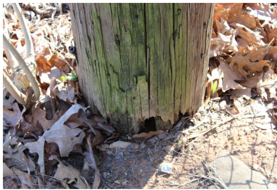
FIGURE 1.3: Photograph of visible symptoms of decay in a pole near the ground line
