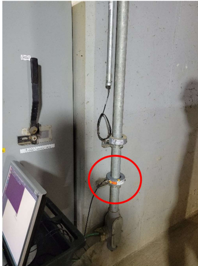
FIGURE 3.3: RF-CT (marked in red) connected to the neutral ground.
