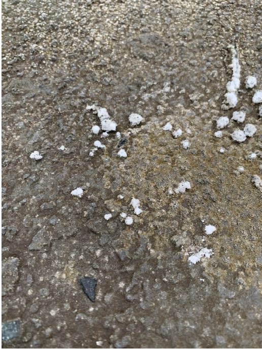
Figure 3.9. Surface salting observed on 10/10/2019.
