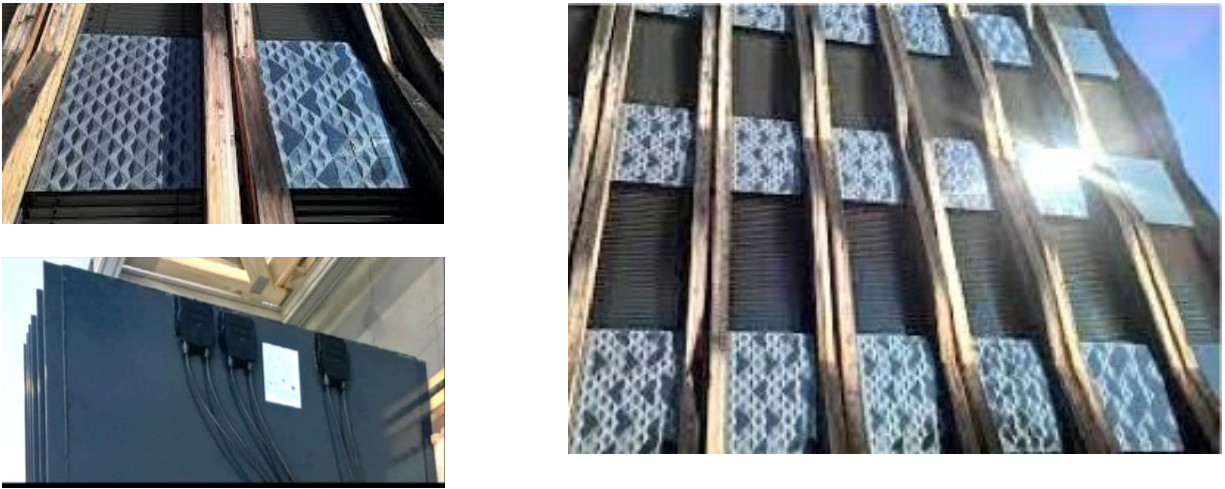
Figure 5: Partial shading on PV modules of Z3 building of Ed. Züblin AG in Stuttgart, Germany. Source: ( Kuhn et al. 2021 )
