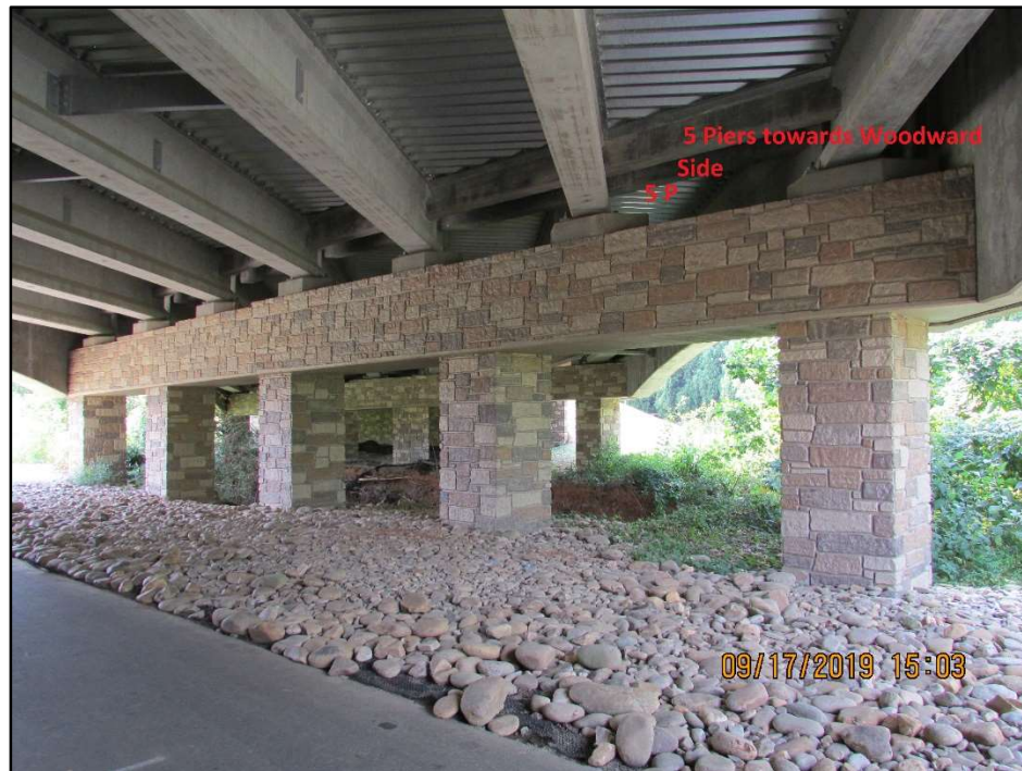
Figure A-1 Road bridge (End Bent 2- 5 piers)
