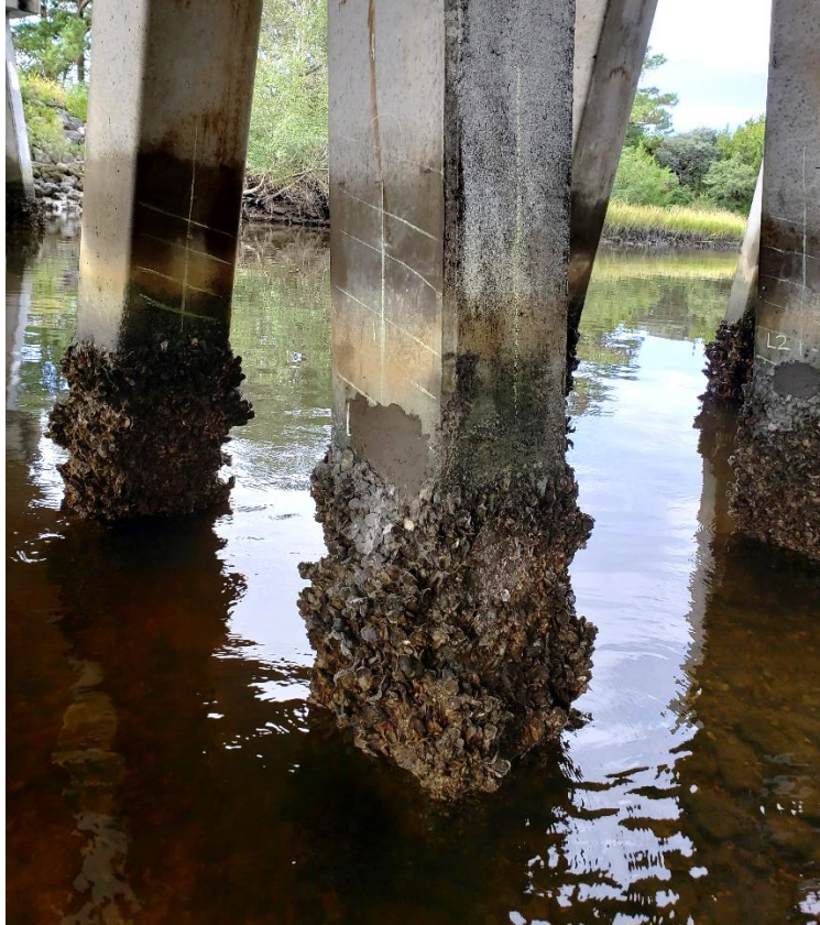
Figure 5.2: Structure 090206 Heavy Fouling Presence (Marine life)
