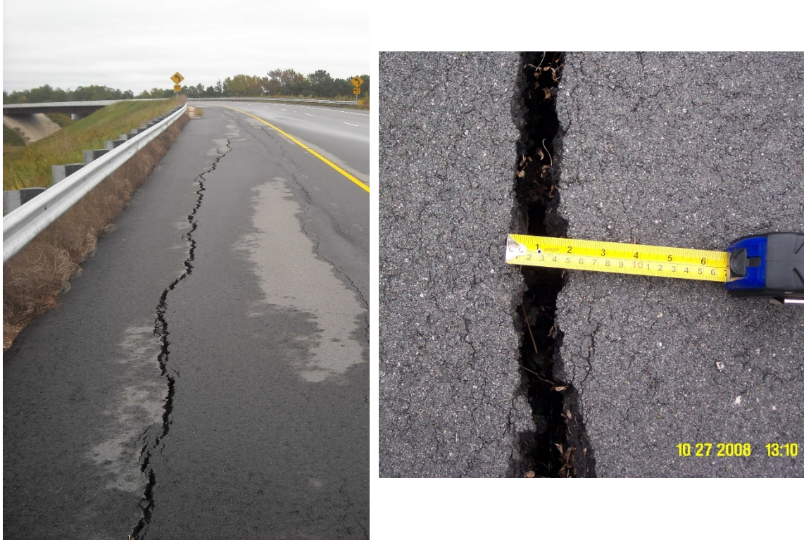
Figure 1.3. Longitudinal cracking at NC I-540 at Davis Drive (Pilipchuk 2008)
