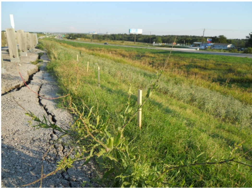
Figure 2.12. Surficial movement and cracked shoulder due to rainfall on U.S. Highway 287, Texas [source: Khan et al. 2015]
