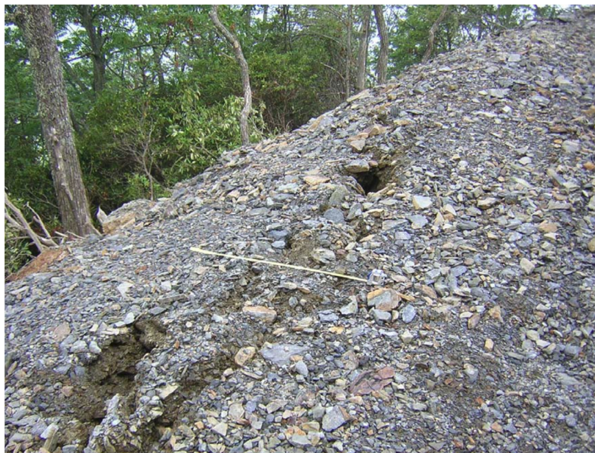
Figure 2.10. View of cracks in embankment, Haywood County, North Carolina (source: NCGS 2006)
