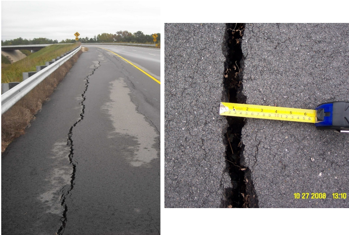
Figure 2.8. Longitudinal cracking on NC I-540 at Davis Drive (Pilipchuk 2008)
