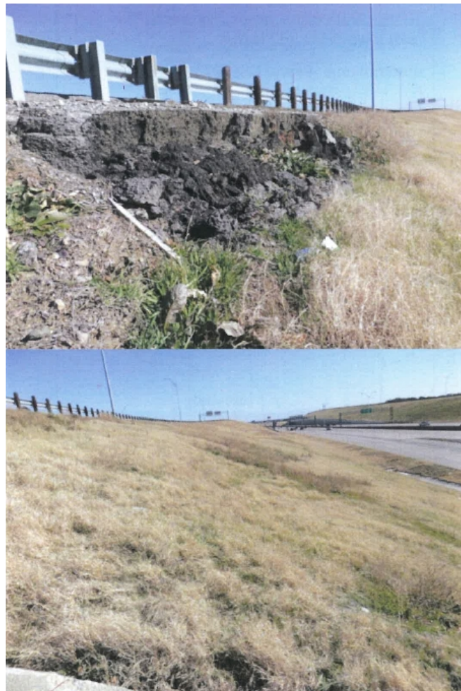
Figure 2.18. Failure of the SH-183 slope (Hossain et al. 2017)
