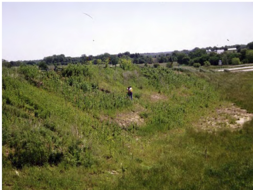
Figure 2.14. South side of embankment at I-70 Emma field showing slide areas S1 (left), S2 (center), and S3 (right) (from Loehr and Bowders 2007)
