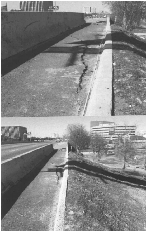
(a) shoulder crack and surficial movement
