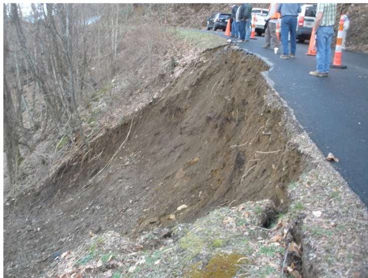
Figure 2.11. Embankment failure from the shoulder of roadway (Appalachian Landslide Consultants 2013)
