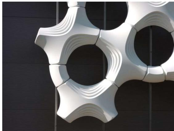
Figure 3: Prototype of façade module for Manuel Gea González Hospital
