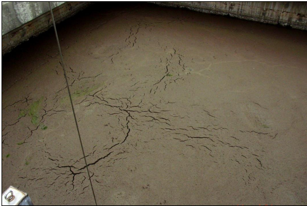
Figure 4.1: Typical Layer of Floating Sludge at 12-Day SRT
