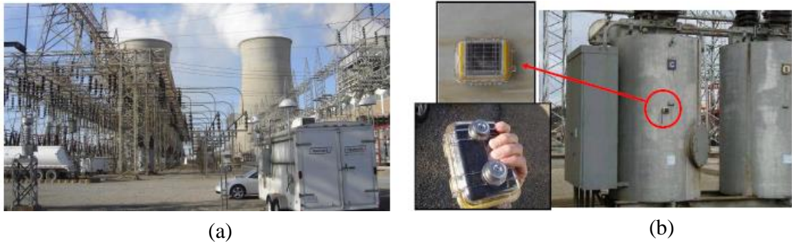
Figure 1.2: (a) Cross-section of the Paradise substation where the ParadiseNet was deployed. (b) a wireless sensor node for monitoring circuit-breakers. [68]
