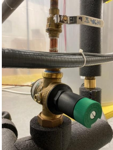
Figure 11: Pressure Reducing Valve for MISAHP System Water Piping
