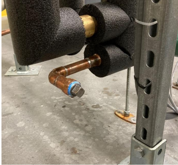
Figure 13: Future Installation Point for Source-Side Expansion Tank
