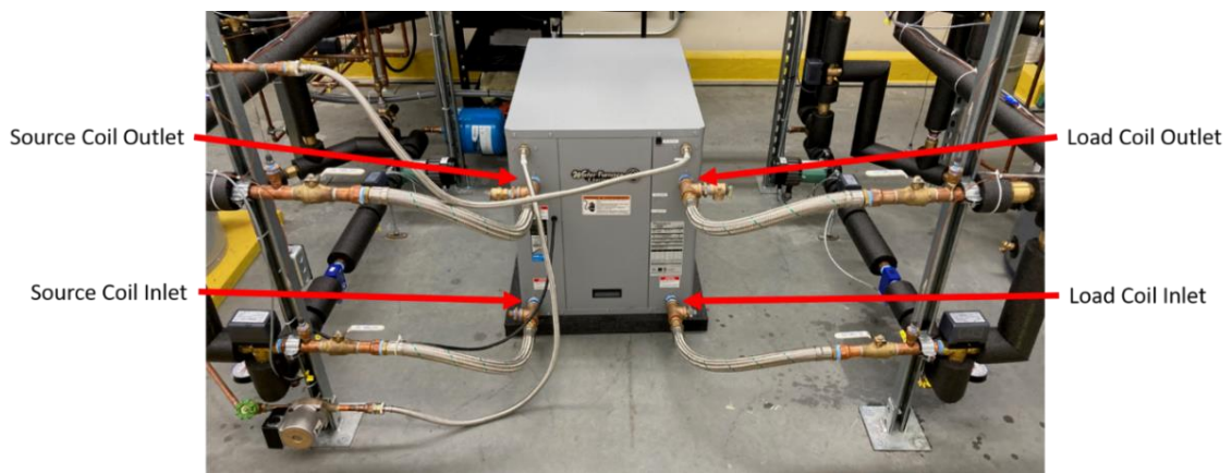
Figure 2: Water-To-Water Geothermal Heat Pump
