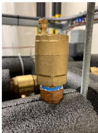
Figure 14: Mechanical Air Vent
