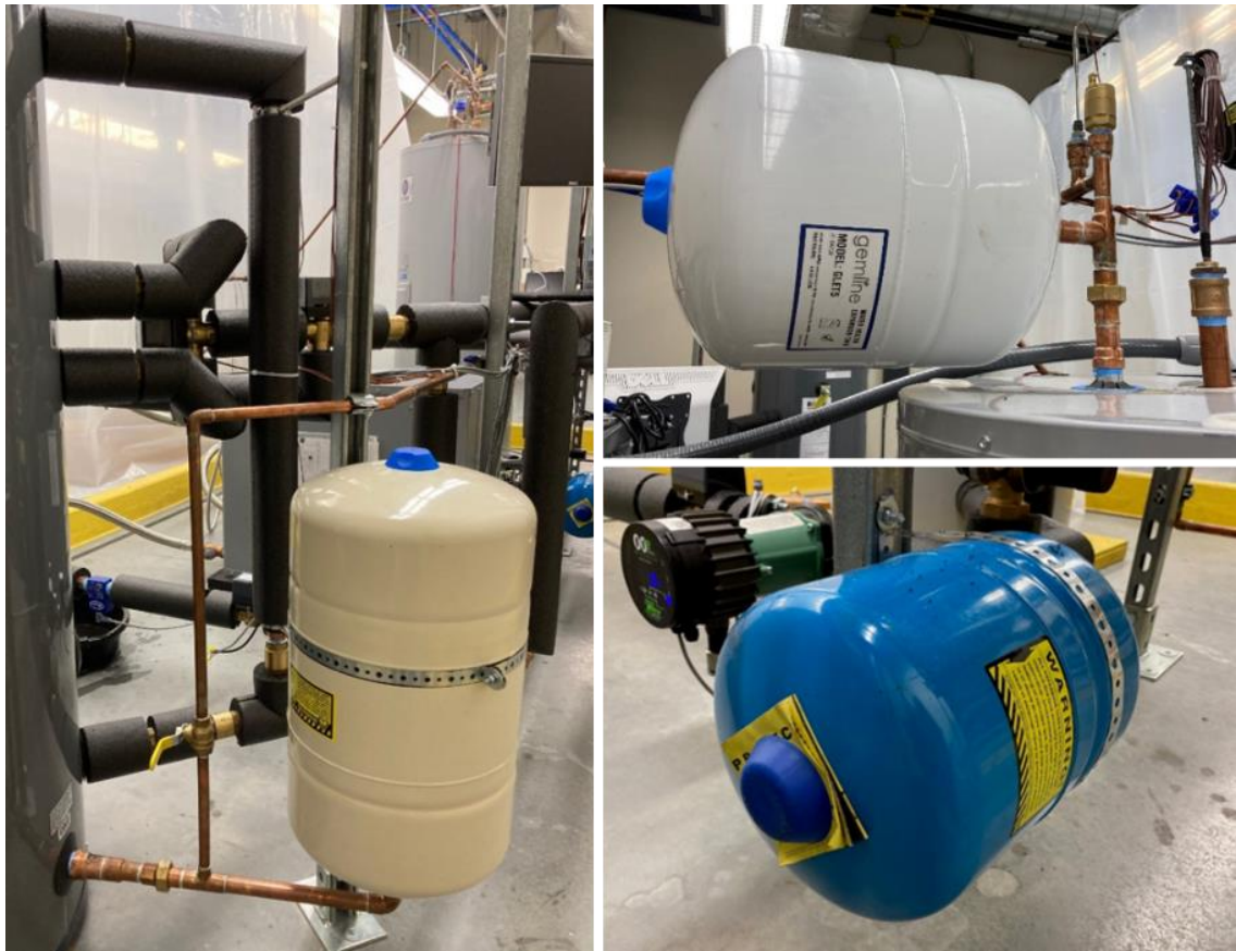
Figure 12: Expansion Tanks -Buffer Storage (left), DHW Tank (top right), Load-Side (bottom right)
