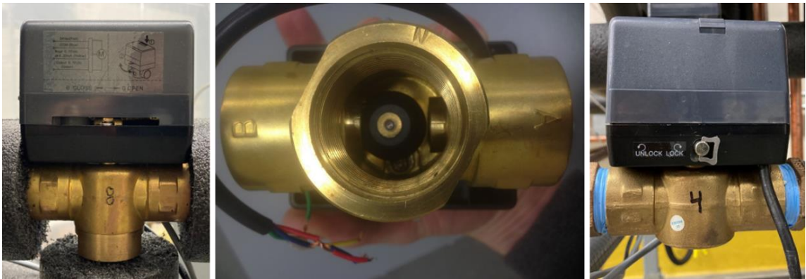
Figure 16: Electronic Valves - 3-way Valve (left), Lever-arm, Stopper, A/B Port Designations (center), and 2-way Valve (right)
