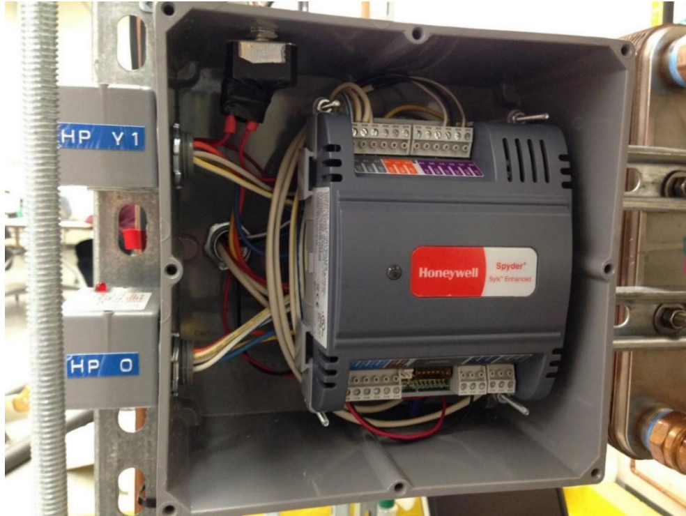
Figure 5: Relay Controller and Relays
