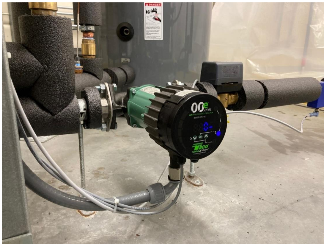
Figure 20: Variable Speed Circulation Pump
