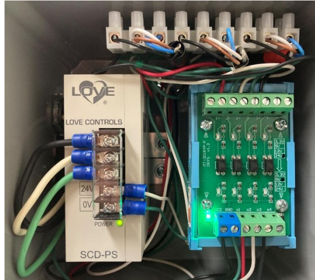
Figure 32: Flow Meter 24VDC Power Supply and Optocoupler for Pulse Signal Voltage Conversion
