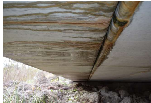
Figure A1.40. Underside of Exterior Cored Slab; Note the Significant Efflorescence.
