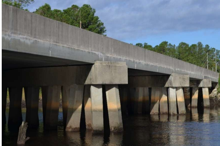
Figure 3.18. Efflorescence at High Tide Line on all Piers.
