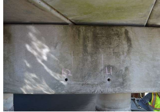
Figure A1.36. Location of Powder Samples on Interior Face of Interior Bent.
