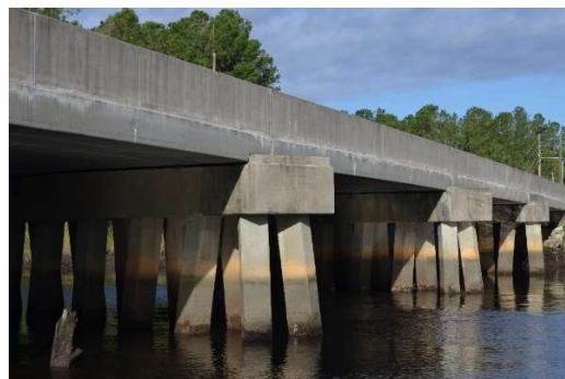
Figure A1.25. Interior Bent Caps and Piers; Notice The Identical Staining on All Piers Showing High Tide Location.
