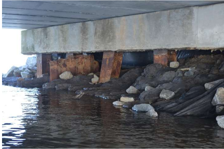
Figure 3.27. Heavily Corroded Interior Bent Steel Piles.
