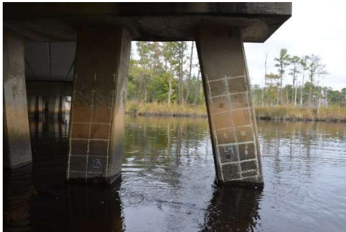
Figure A1.23. Testing Grid Location on Piers with Powder Sample Locations Identified.
