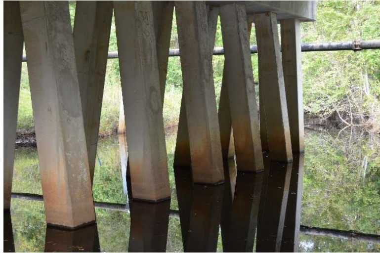
Figure 3.16. Efflorescence within Splash Zone of Piers.
