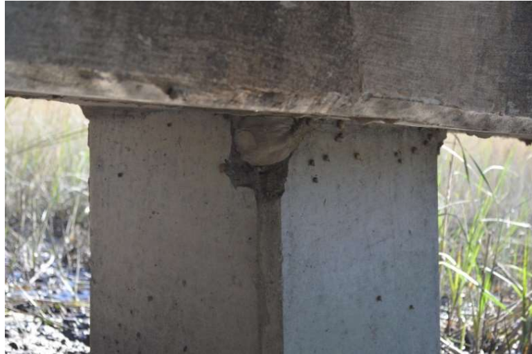
Figure 3.21. Spalled Section at Pier to Bent Cap Connection.
