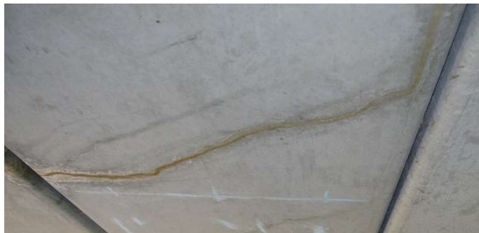
Figure 3.13. Example of Large Cracked and Repaired Section on Underside of Cored Slab.
