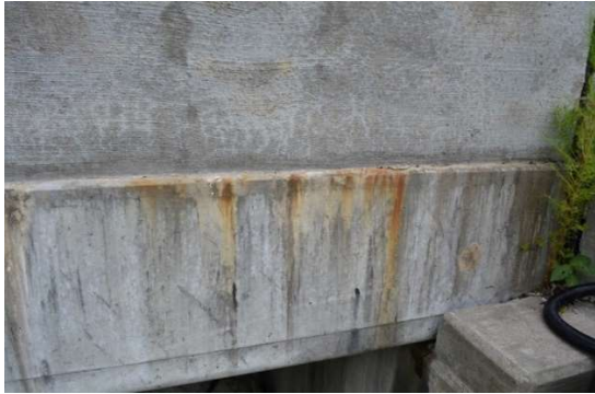
Figure A1.8. Efflorescence on Side Face of Cored Slab at Southwestern Side of End Bent 1.
