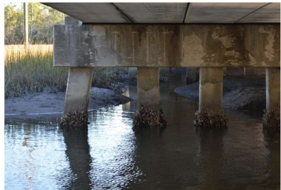
Figure A1.29. Testing Grid For iCOR; Notice the Significant Shell Buildup on The Piers.
