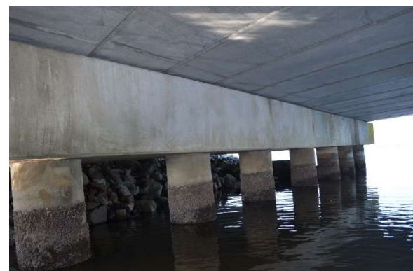
Figure A1.38. Interior Cap with Piers. Note the Significant Barnacle Buildup at The High Tide Line.
