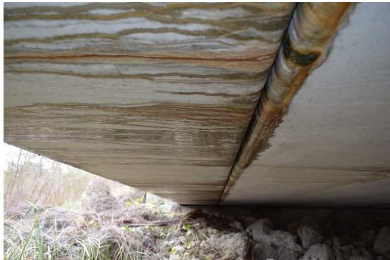
Figure 3.30. Efflorescence on Underside of Cored Slab.
