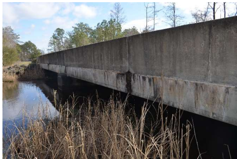
Figure 3.24. Efflorescence Staining on Side of Exterior Cored Slabs.
