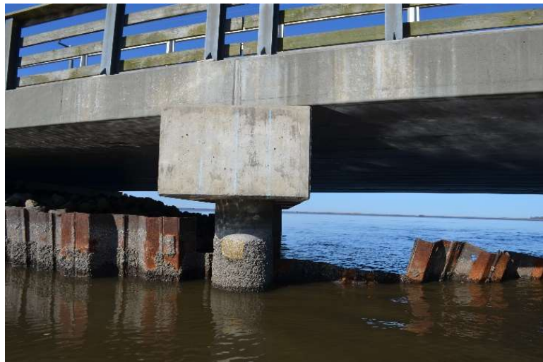
Figure 3.28. Heavily Corroded Steel Sheet Piles.
