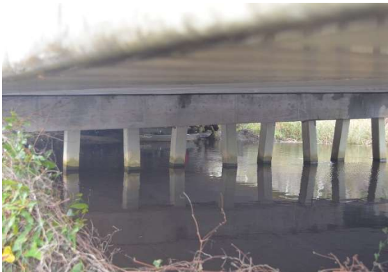
Figure A1.39. Interior Cap with Piers; Note the Drainage Patterns on Right Side of Cap.
