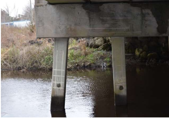
Figure A1.41. Location of Multiple iCOR Test Grids and Powder Sample Sites.
