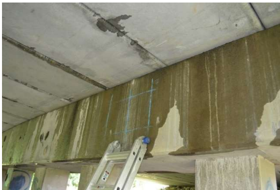
Figure A1.6. Location of iCOR Test Grid and Powder Sample Site on Face of Interior Bent.
