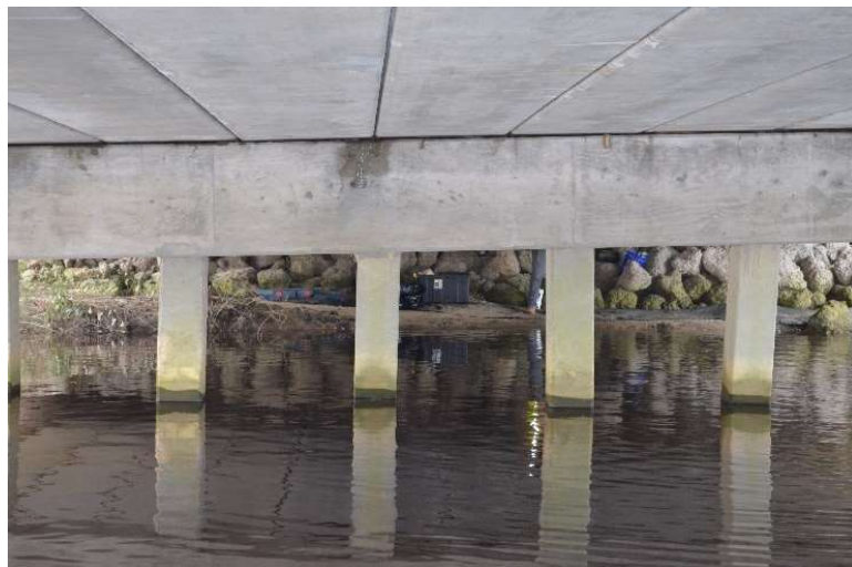
Figure 3.31. Efflorescence within splash zone on interior bent piles.
