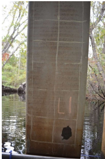
Figure A1.18. Location 1 Of iCOR Testing Grid and Powder Sampling Location.
