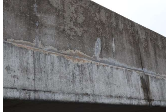
Figure A1.42. Exterior Face of Concrete Barrier Wall; Note the Cracking and Staining.
