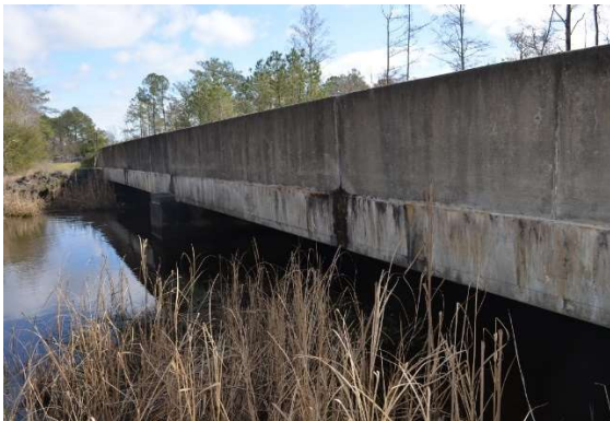
Figure A1.33. Side Face of Cored Slabs. Note the Staining on Right Side of Image.
