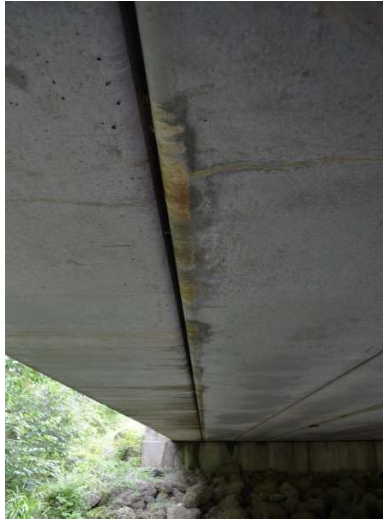
Figure A1.10. Efflorescence on Underside of Cored Slab.
