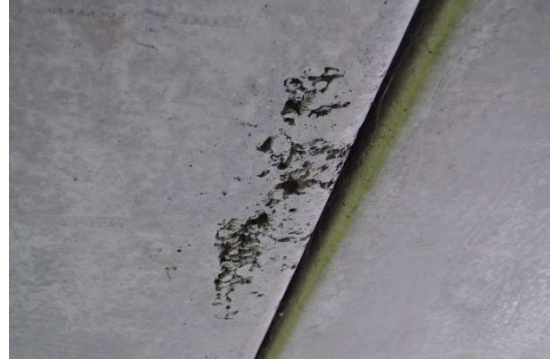
Figure A1.9. Deep Section of Honeycombing on Underside of Cored Slab.
