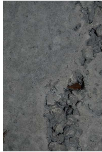
Figure A1.11. Close-Up of Honeycombing (Shown in Figure A1.9); Note Exposed Rebar.
