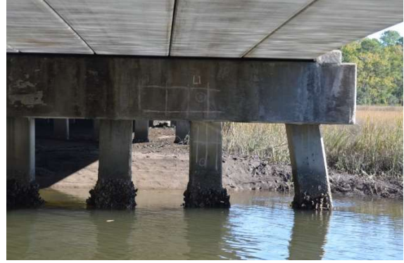
Figure A1.27. Testing Grid For iCOR And Powder Sample Locations 1 And 2.
