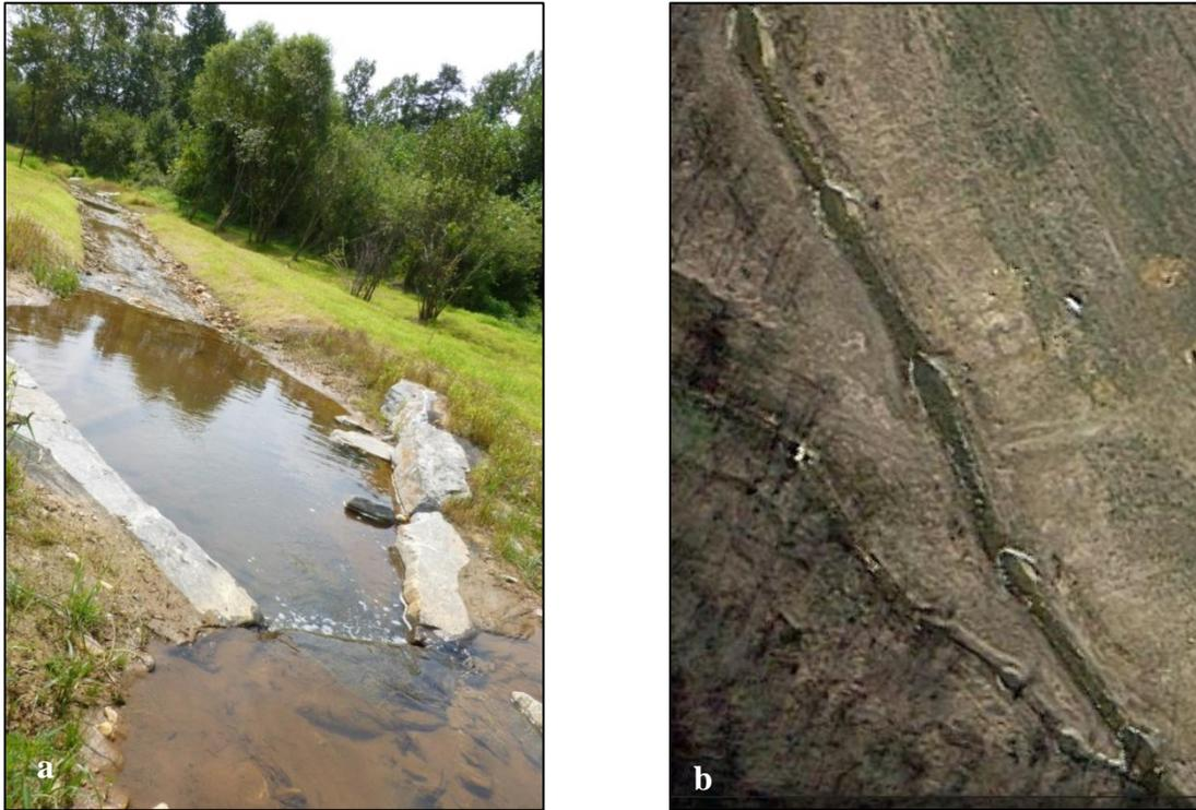
Figure 4: Natural channel design stream restoration approach. a) A boulder cross vane structure in the restored stream channel, creating a riffle, step, pool sequence. b) Aerial view of cross vane structures in the restored stream channel.
