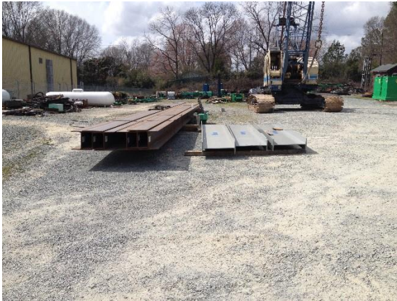
a.) Piles and beam for reaction frame, steel beams for reaction piles provided by Skyline Steel, LLC
