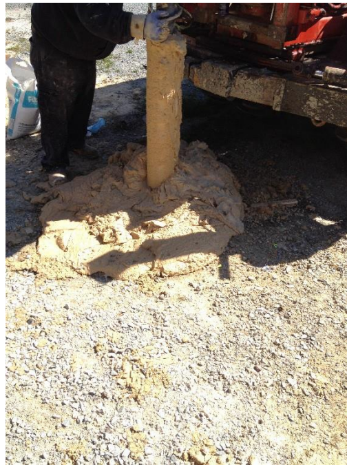
c.) Soft soil encountered during SPT boring
