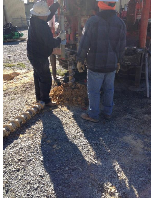
b.) Performing SPT boring
