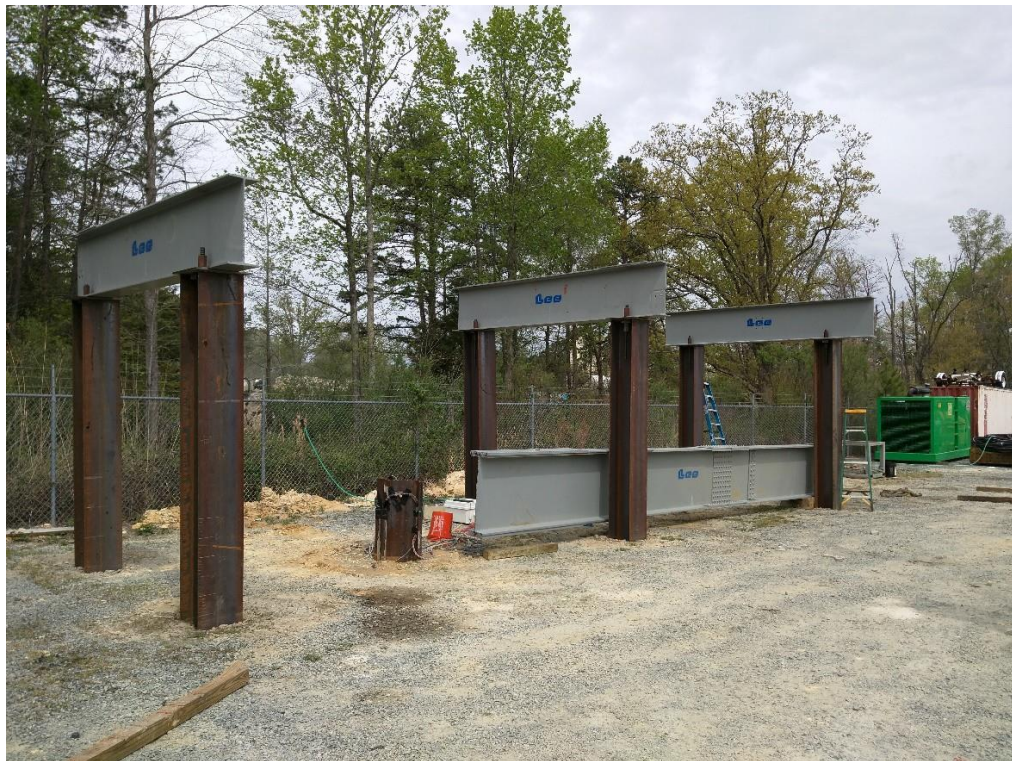
Figure C-15. Image of transfer beams bolted to reaction frame, installation of reaction pile and placement of transfer beams courtesy of ICE
