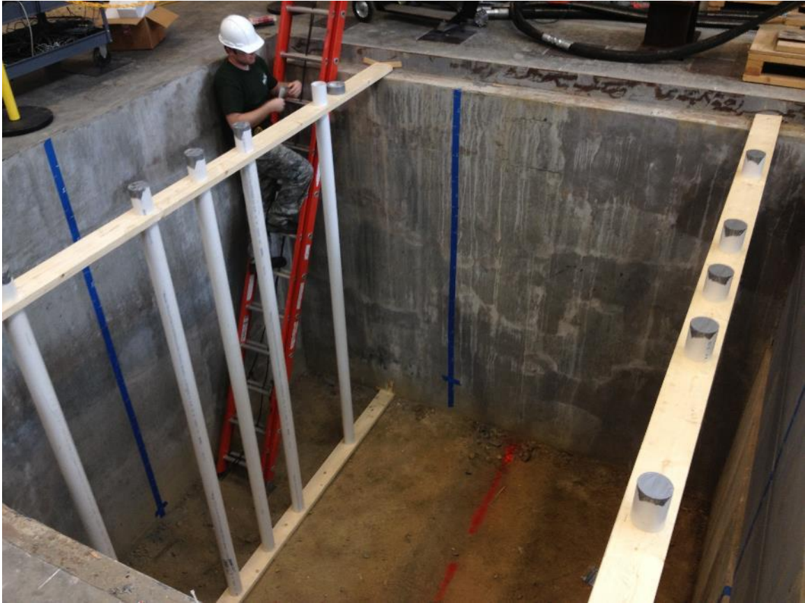
Figure 3-1. Geotechnical test pit at UNCC
