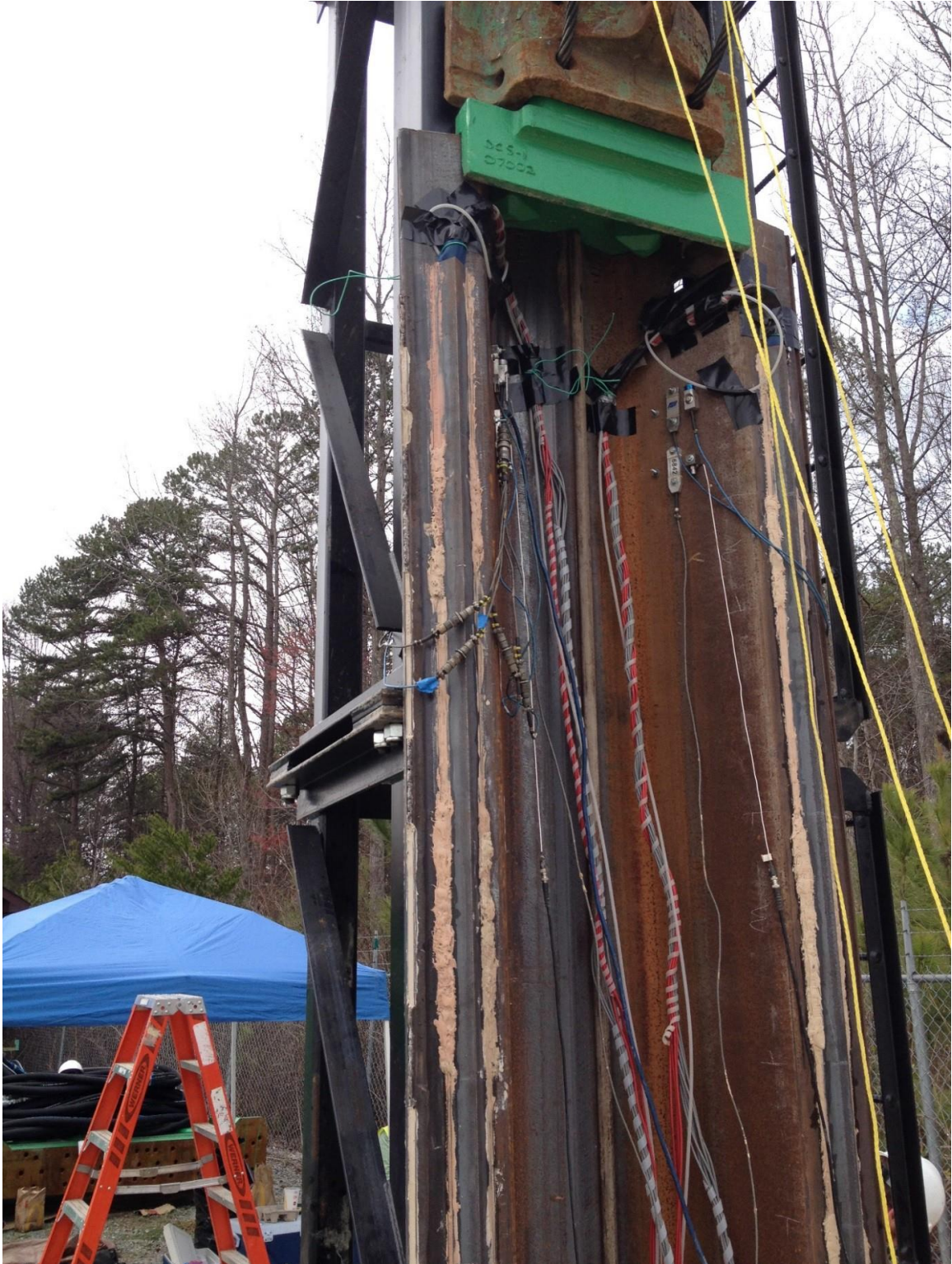
Figure C-11. Image of PDA instrumentation during impact driving of sheet piles at ICE field site, PDA testing performed in conjunction with GRL
