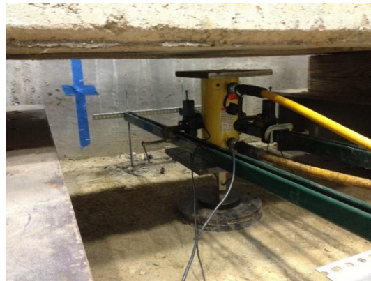
(c) Close up of plate load test setup
