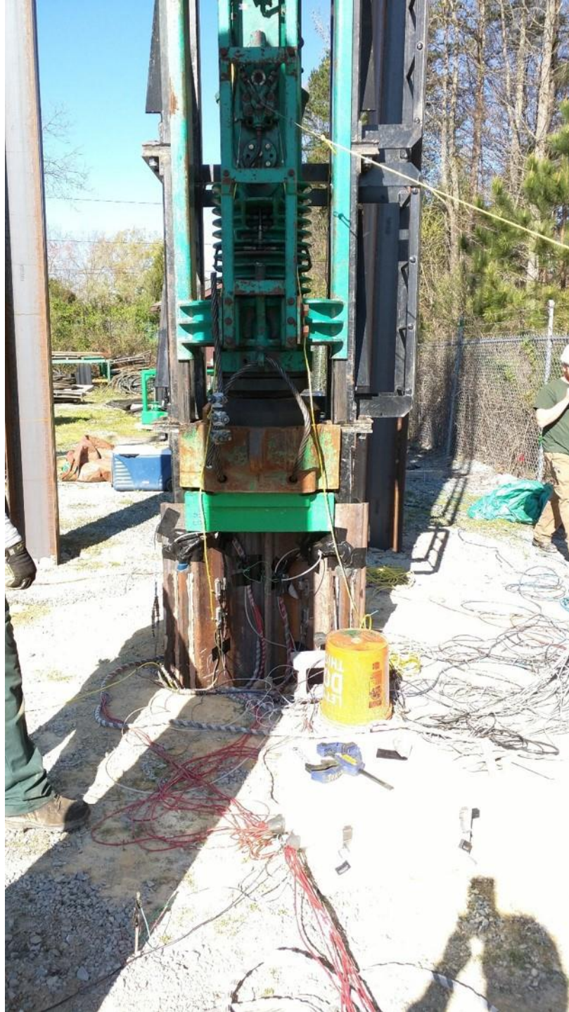
Figure C-12. Photo of impact driving and PDA instrumentation during restrike testing of sheet piles at ICE field site
