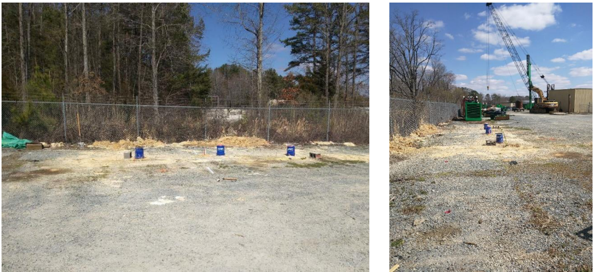
Figure C-2. Field site after site characterization geotechnical testing
