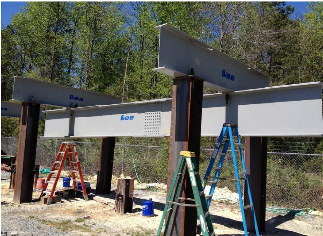
Figure C-16. Images of assembled reaction frame and driven H-pile for load testing
