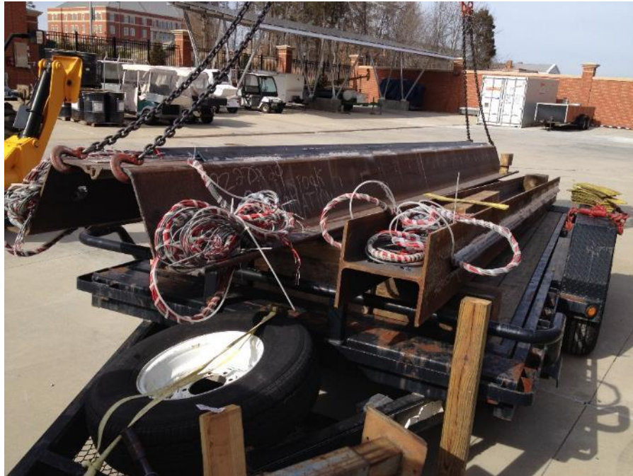
Figure 4-13. Image of test piles prior to installation
