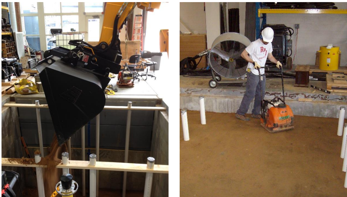
Figure 3-3. Images taken during backfilling of geotechnical test pit at UNCC
