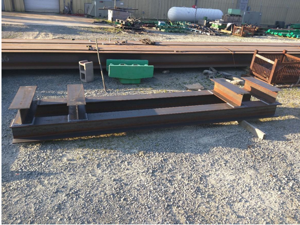
Figure C-14. Image of steel beams used for piles and installation guide frame constructed by ICE for reaction pile driving
