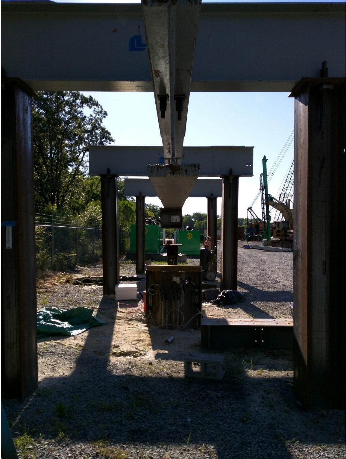
Figure C-17. Side view of test piles and reaction frame at ICE field site
