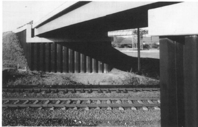
a.) Image of Humber road bridge
