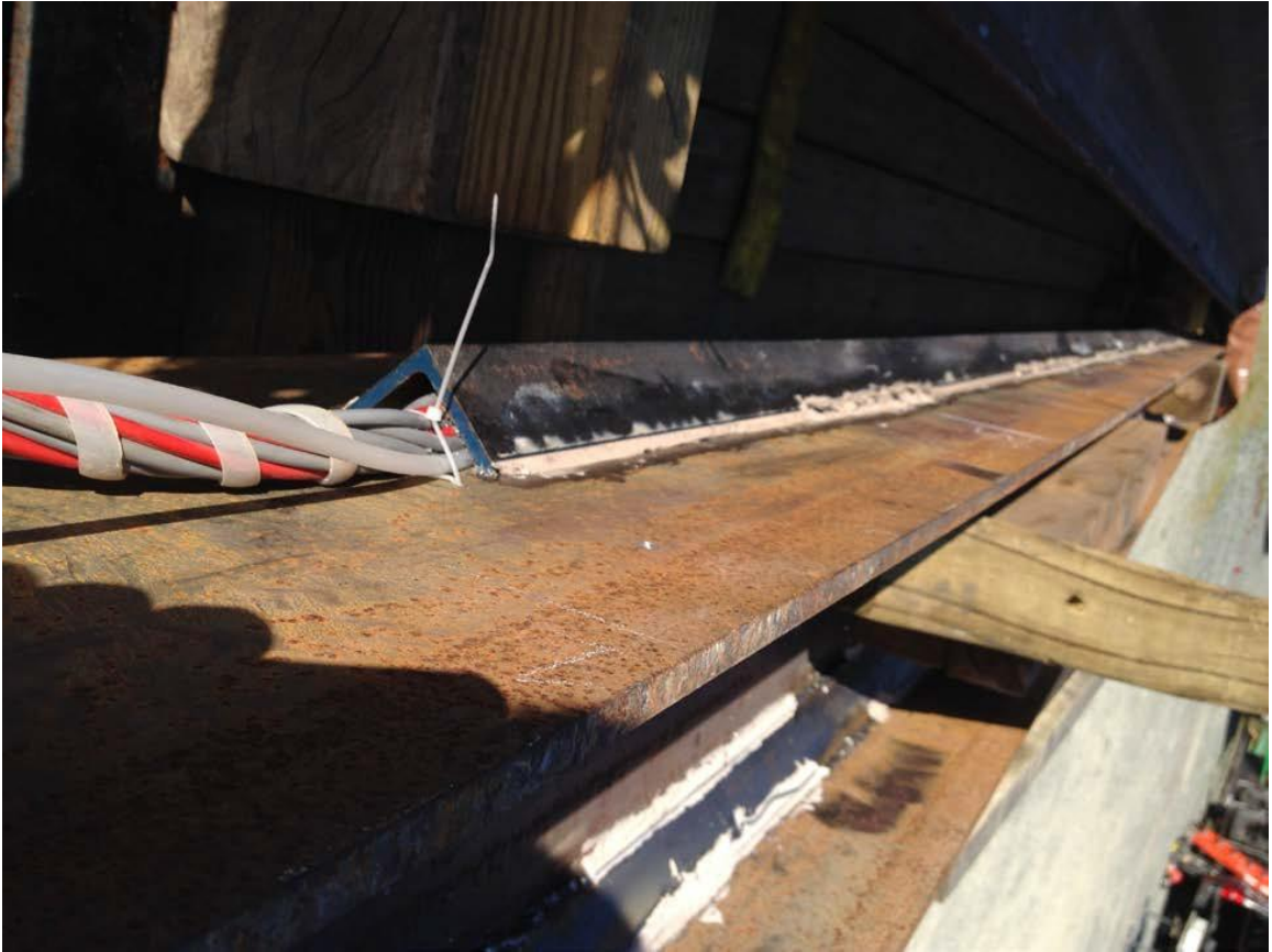
Figure C-9. Image of instrumented H-pile for field load testing program
