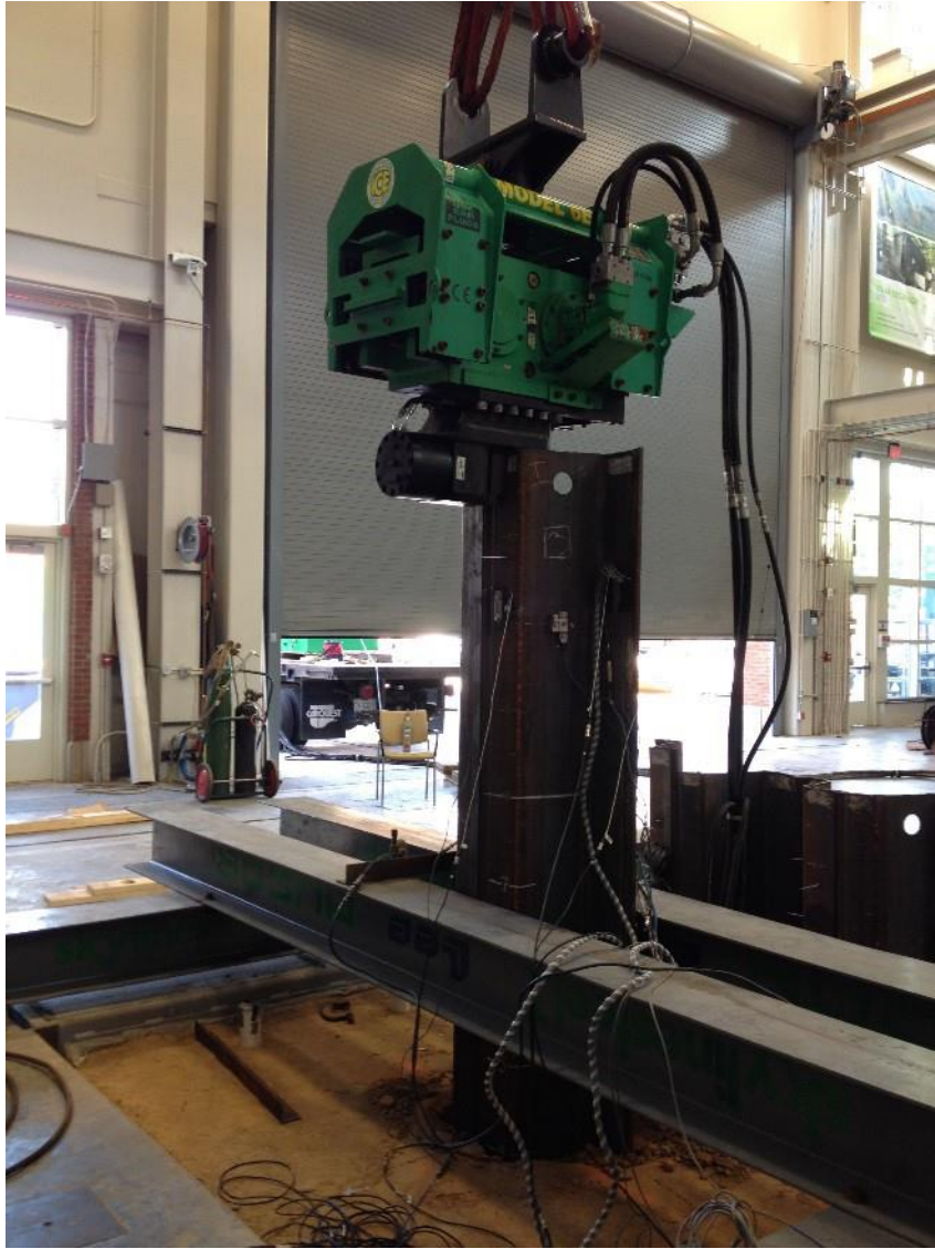
Figure B-16. Driving sheet pile with ICE Model 6E vibratory hammer
