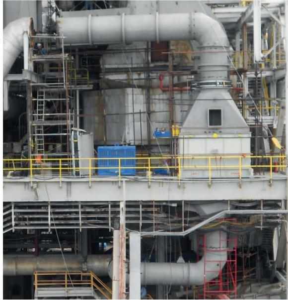
Figure 1.7: Installed Package Rotary Air preheaters on a power plant site [35]
