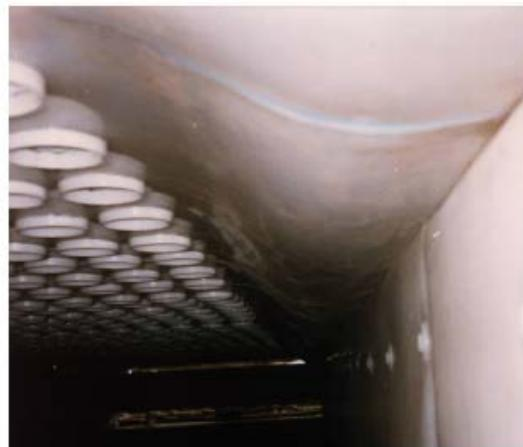
Figure 2.14: Modular Design of GAGAVO Heat Exchanger with PTFE Tubes. Internal Surface are Lined by PFA Fluoroplastic Sheets [3]
