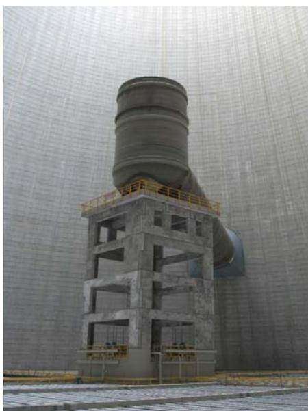
Figure 5.3: Flue gas stack inside a natural draft wet cooling tower [42]
