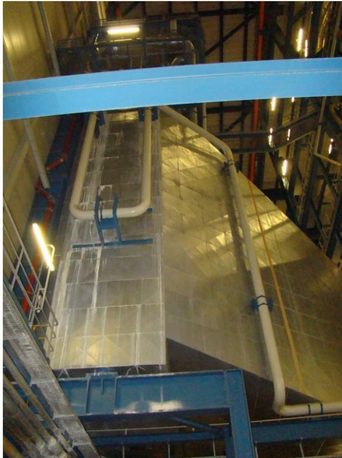
Figure 2.12: Side View of the FGC at Schwarze Pumpe Retrofitted with Corrosion-Resistant Alloy Tubes, October 2008 [3]
