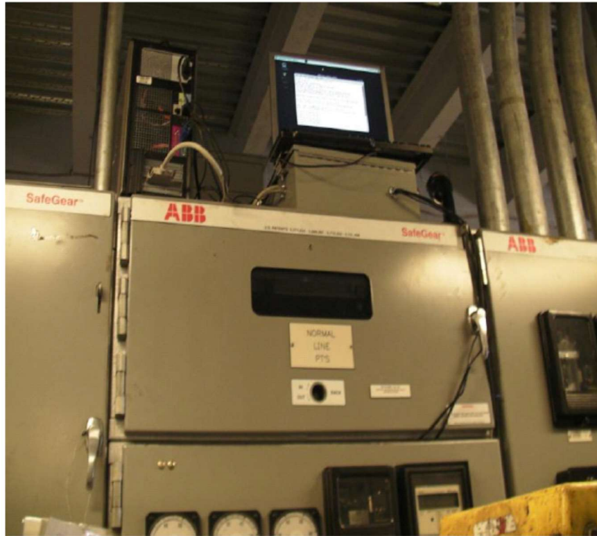
Figure 3.3: Picture of the NILM installation. The NILM computer and box are at the top of the crusher panel.
