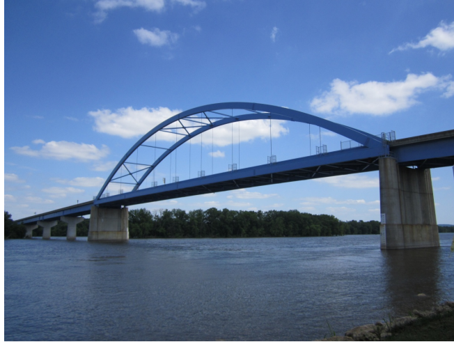
Figure 3: Steel tied arch bridge serving as case study structure
