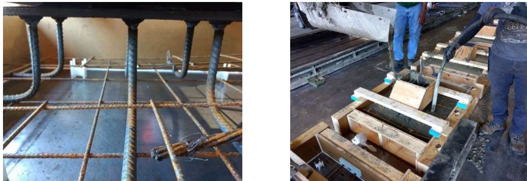
FIGURE 4.9: (a) Interior view, bent bars. (b) Pouring and vibration of specimens.
