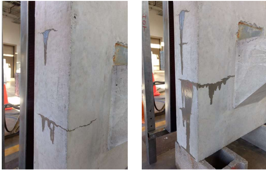
FIGURE 4.51: Specimen N3: Formation of tiered cracking.
