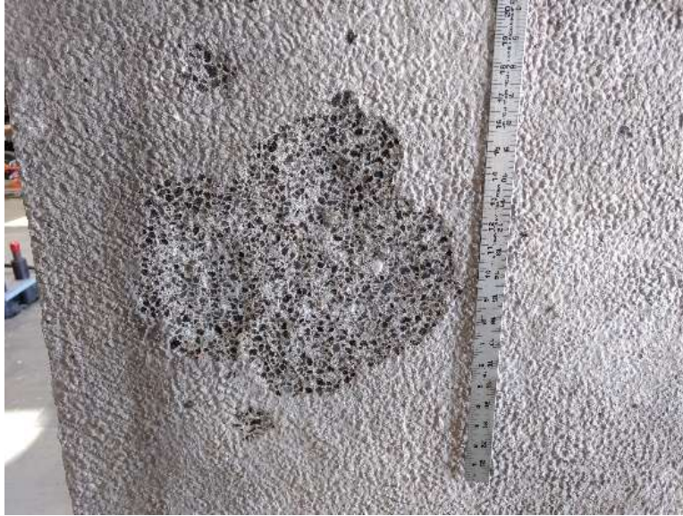
FIGURE 4.72: Spalling damage of specimen L10.
