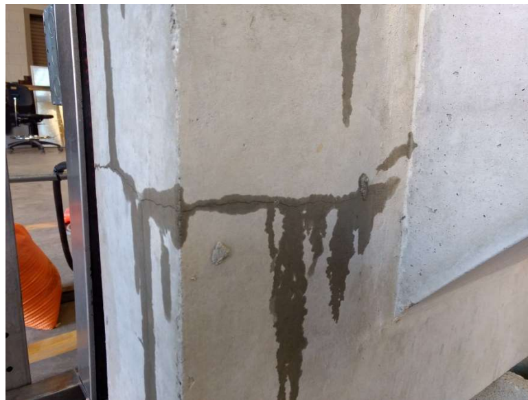
FIGURE 4.63: Specimen N6: Cracking and leakage towards corbel and wall interface.
