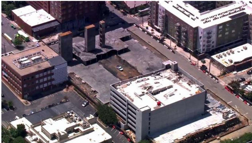
FIGURE 4.3: Post fire, remaining stairwells and parking deck (Wtvd, 2017).
