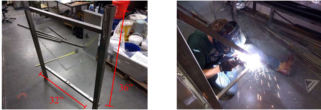
FIGURE 4.12: (a) Frame construction progress. (b) Welding of cross bars.
