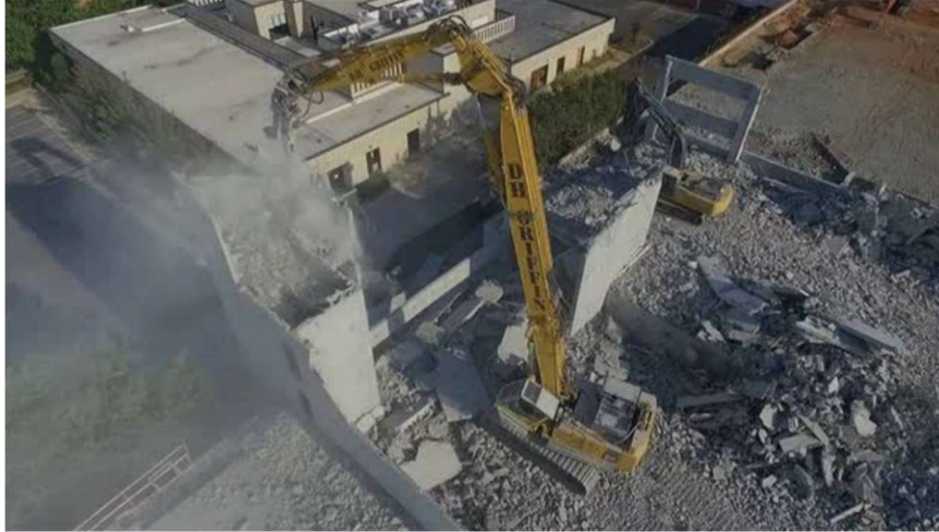
FIGURE 4.4: Demolition of adjacent parking deck (Wtvd, 2017).
