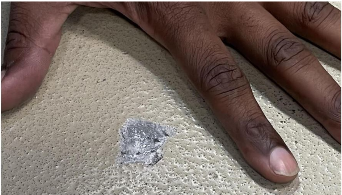
Figure 6.11: Shallow chip in floor approximately 25 mm in diameter.
