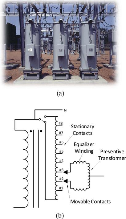
**FIGURE 1.** (a) SVRs in the substation. (b) Configuration of the conventional SVR.
