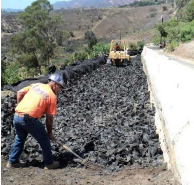
Figure 2.29: Type B TDA utilized in roadway construction (CalRecycle, 2015)
