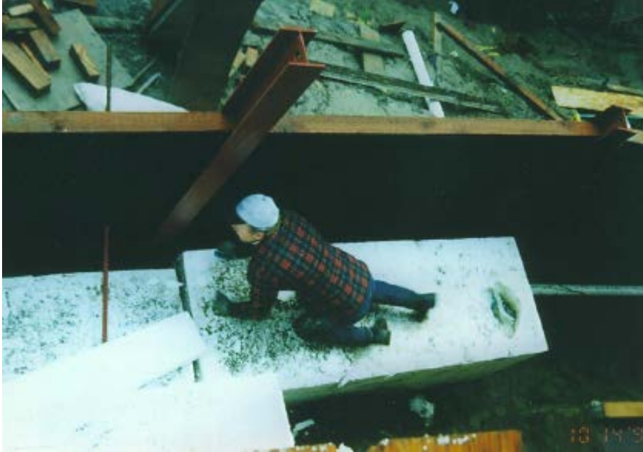
Figure 2.16: EPS Geofoam block field installation (Mann and Stark, 2007)
