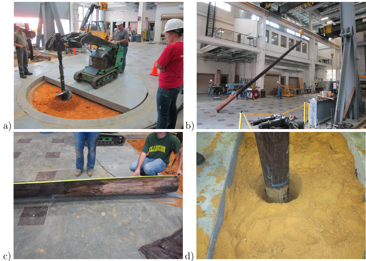
FIGURE 3.2: Installation of timber distribution poles in experimental test bed: a) augering holes with skid steer, b) lifting poles with overhead crane c) measuring pole dimensions and marking pole, d) installing pole to original depth of embedment
