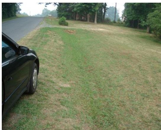
d) Road with ditches flowing diffusely e) Road without ditches flowing diffusely
