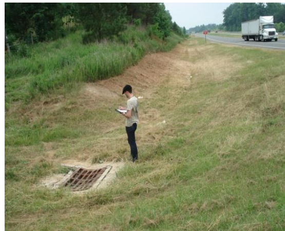
a) Road with curbs connected with drains b) Road with ditches connected with a drain
