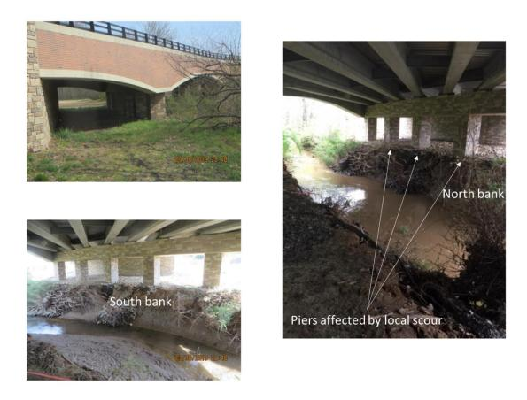
Figure 3-3 Snapshots of Phillips Road Bridge (on 03/30/2019)
