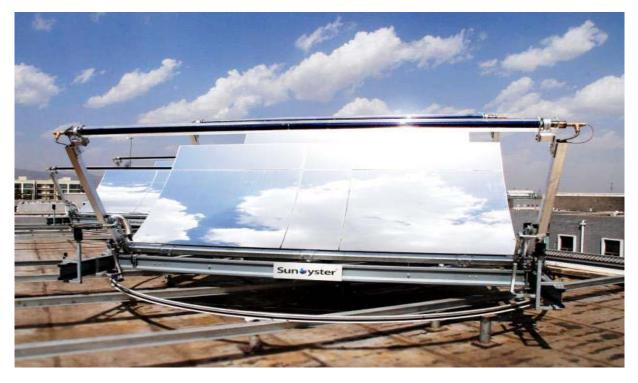
Figure 2-5: Concentrating PVT collectors manufactured by Sunoyster (n.d.)
