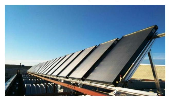
Figure 2-3: Covered PVT collectors manufactured by Endef (2020)
