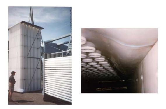
Figure 2.14: Modular Design of GAGAVO Heat Exchanger with PTFE Tubes. Internal Surface are Lined by PFA Fluoroplastic Sheets [3]
