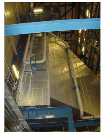
Figure 2.12: Side View of the FGC at Schwarze Pumpe Retrofitted with Corrosion-Resistant Alloy Tubes, October 2008 [3]
