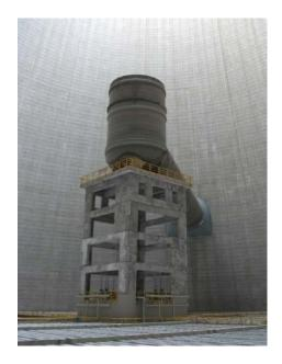
Figure 5.3: Flue gas stack inside a natural draft wet cooling tower [42] (Courtesy Hamon Thermal GmbH Pvt. Ltd.)
